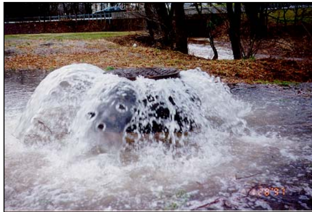
Figure 1.4.6-2 Overflowing Manhole Near a Stream
