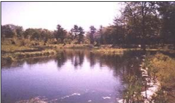
A storm water wetland detains storm water, removes pollutants, and provides habitat and aesthetic benefits (Source: The Bioengineering Group, Inc., no date)
