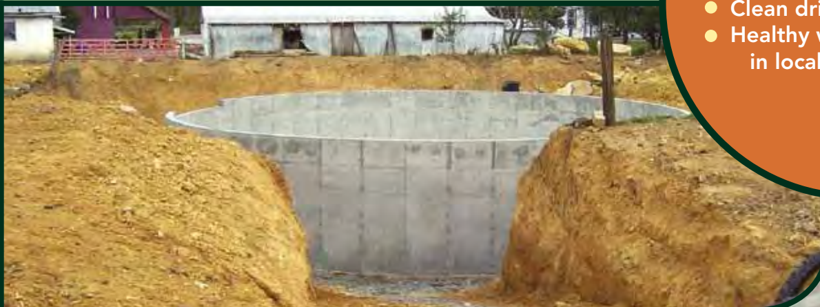
An in-ground liquid manure tank during construction.
