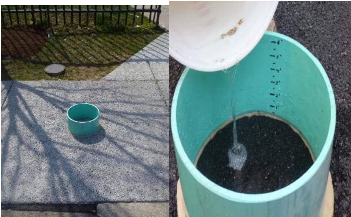
Figure 4-4: Pervious Paving Infiltration Testing Procedure
