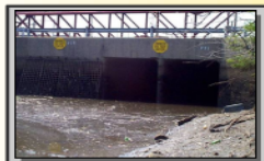
#5 F21 805 MG/yr. Frankford Creek Walding Street northwest of Creek Basin Twin outfall 10.5' x 9.5'
