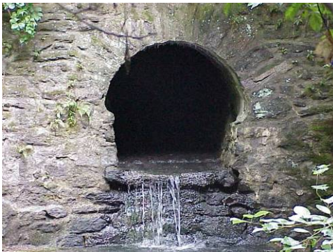
Figure 4.16 Stormwater Outfall
