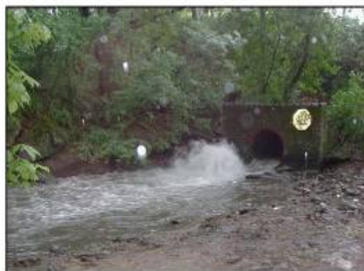
Combined Sewer Overflow at Crescentville in Philadelphia
