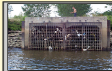
#8 D5 416 MG/yr. Delaware River Magee Street southeast of Milnor Street Twin outfall 11' x 9'
