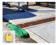
Do extend silt sock 12" beyond trench drain to ensure proper filtering and stable placement.
