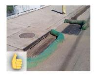
Do direct flow around/away from highway style inlets and trench drains when an inlet filter bag is not feasible.
