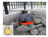
Do completely cover riser with heavy duty plastic (contractor's bag or heavier). Use tape to seal the bag, ensuring no leakage.
