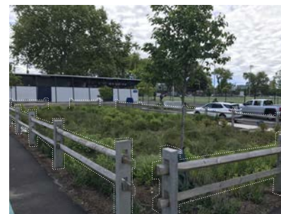
Split rail fencing deters users cutting through the system and protect against cyclists
