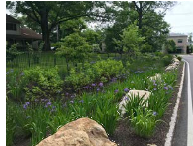
Boulders protect the system from vehicles parking on the edge
