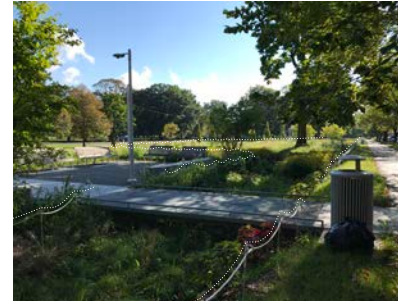
Temporary stake and rope fencing defines the edge while GSI plantings are establishing
