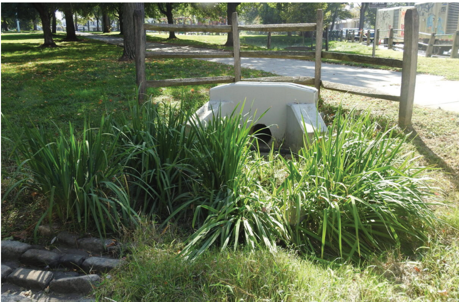
This image showcases how water enters into the rain gardens from the street (the blocks in the lower left), as well as how smaller rain gardens are connected to larger rain gardens via a pipe network (under the sidewalk).
