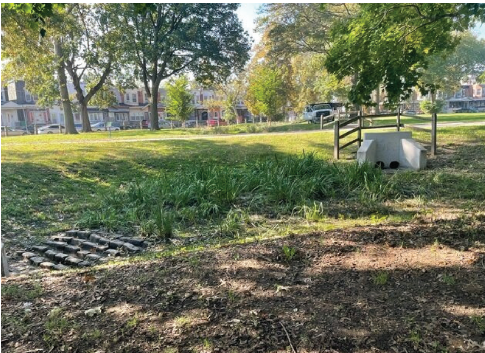
This rain garden manages stormwater runoff from the streets next to the park and is planted with Blue Flag Iris.
