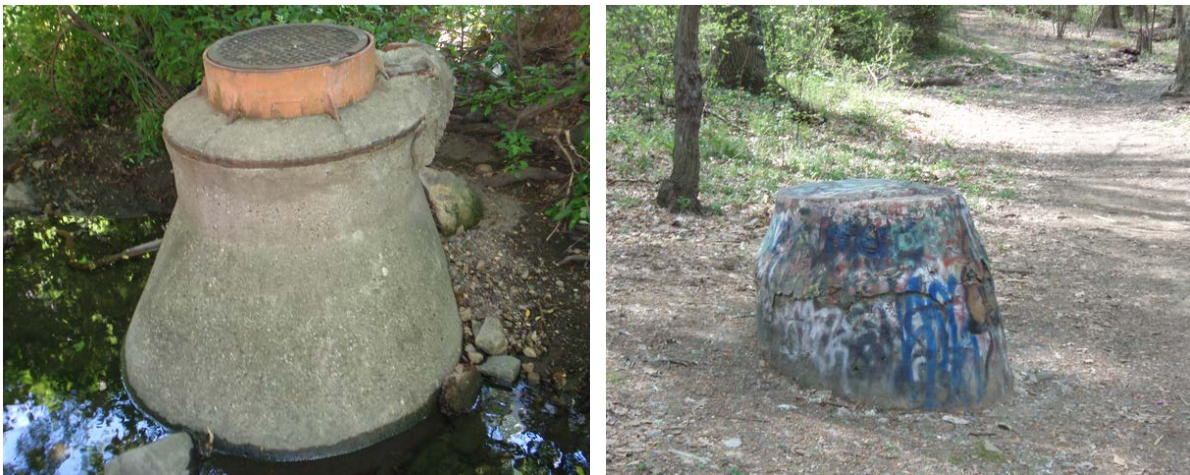
Figure 2-9: Examples of manholes assessed in infrastructure trackdown.
