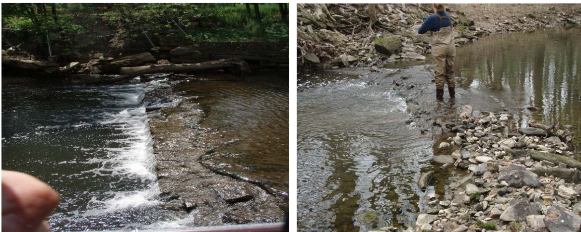
Figure 2-11: Examples of dams assessed in infrastructure trackdown.
