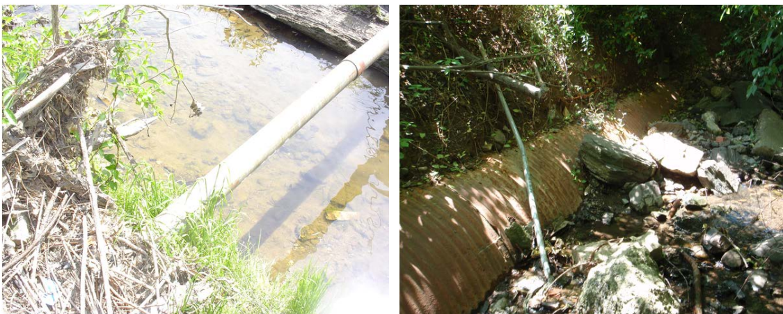
Figure 2-13: Example of a pipe assessed in infrastructure trackdown.
