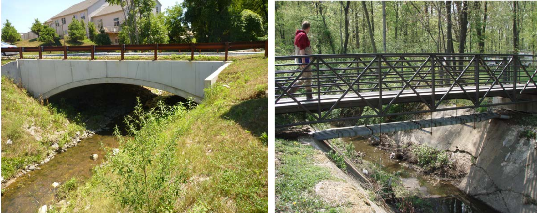
Figure 2-8: Examples of bridges assessed in infrastructure trackdown
