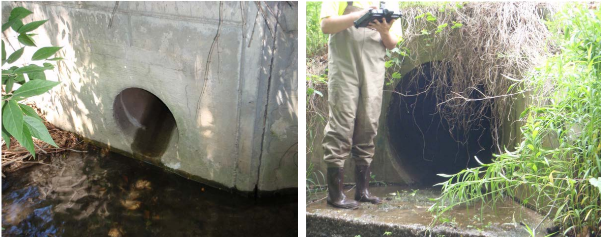
Figure 2-7: Example of an outfall point assessed in infrastructure trackdown
