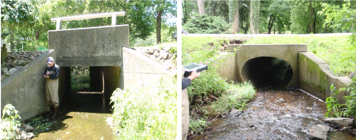
Figure 2-10: Examples of culverts assessed in infrastructure trackdown.
