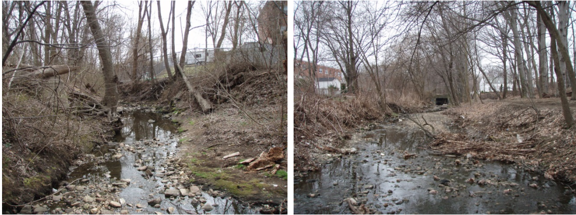
Figure 3- 119: Left- downstream view of PQGR02, Right- downstream view of PQGR06
