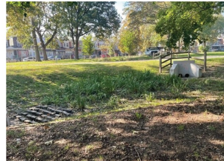
This rain garden manages stormwater runoff from the streets next to the park and is planted with Blue Flag Irises.
