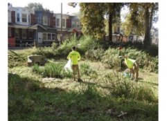
All public GSI systems, including these rain gardens, are maintained regularly for peak functionality and to ensure the health and safety of the site, care-givers, and park users.
