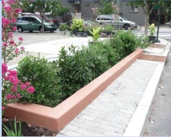
Stormwater Bumpout
