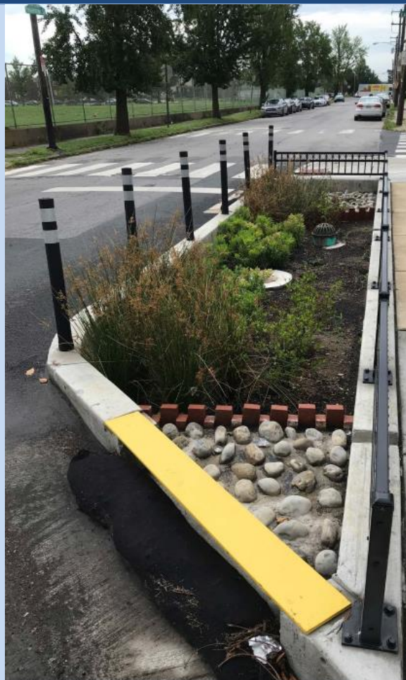
Stormwater Bumpout
