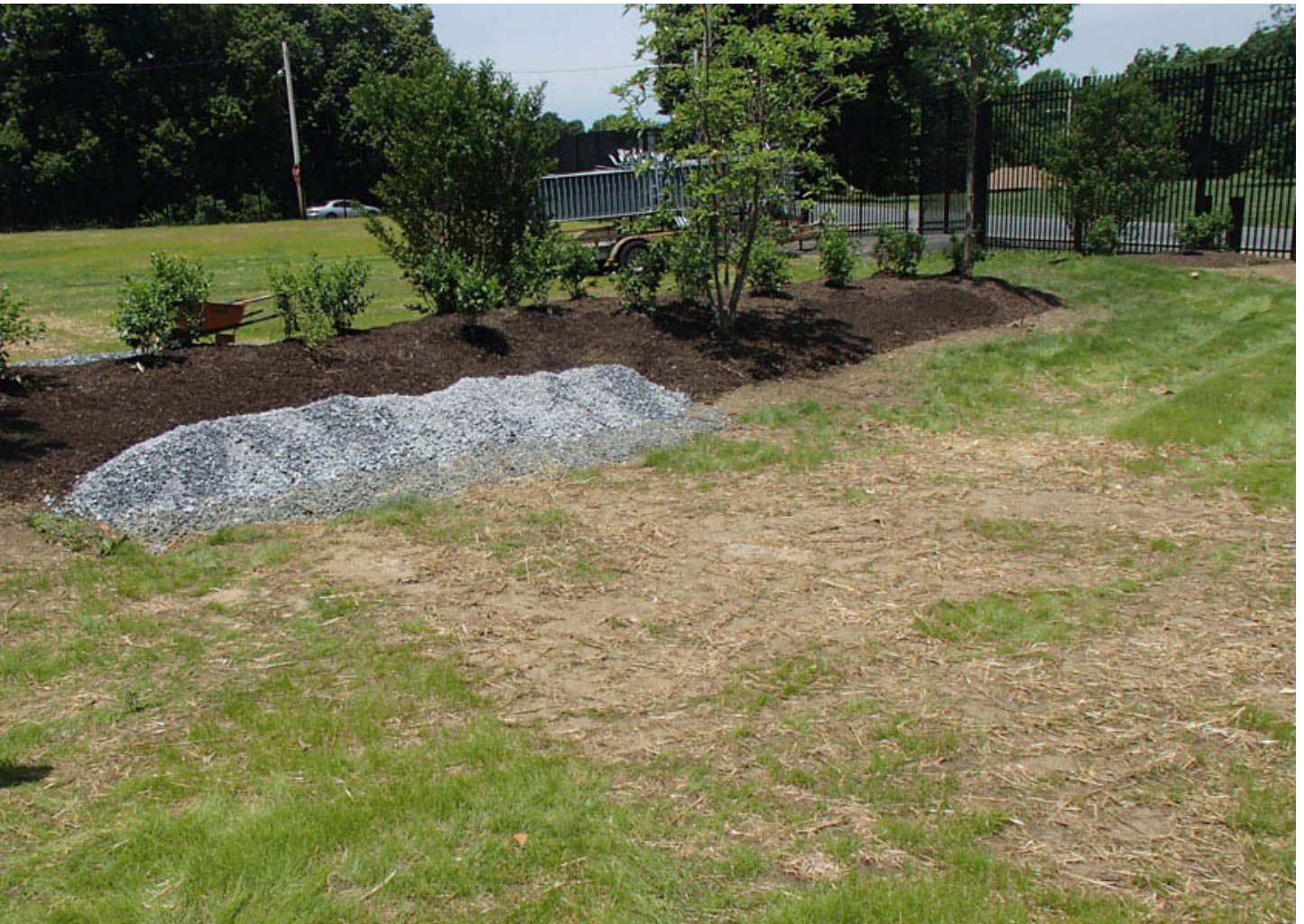
An example of a level spreader in Philadelphia
