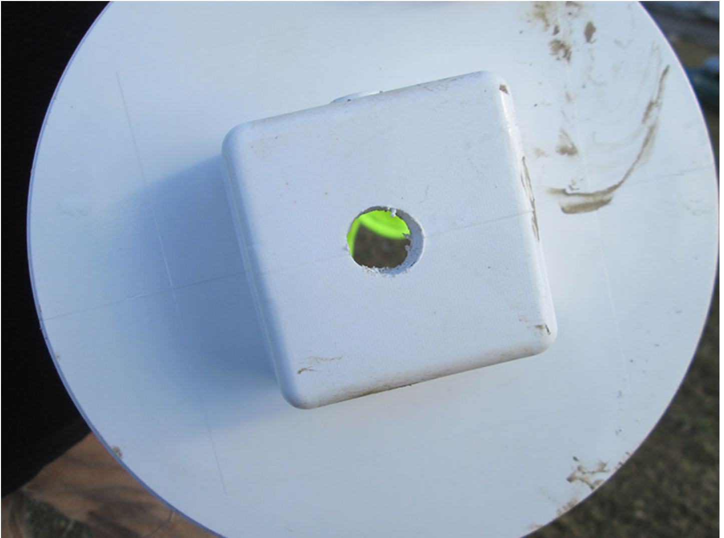
An example of an underdrain orifice in Philadelphia
