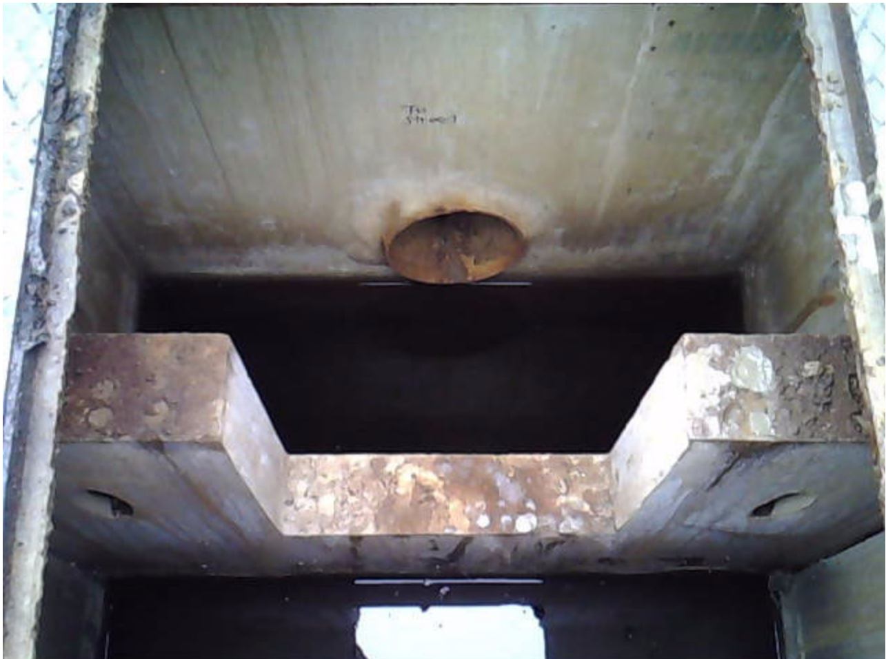
An example of a weir in Philadelphia
