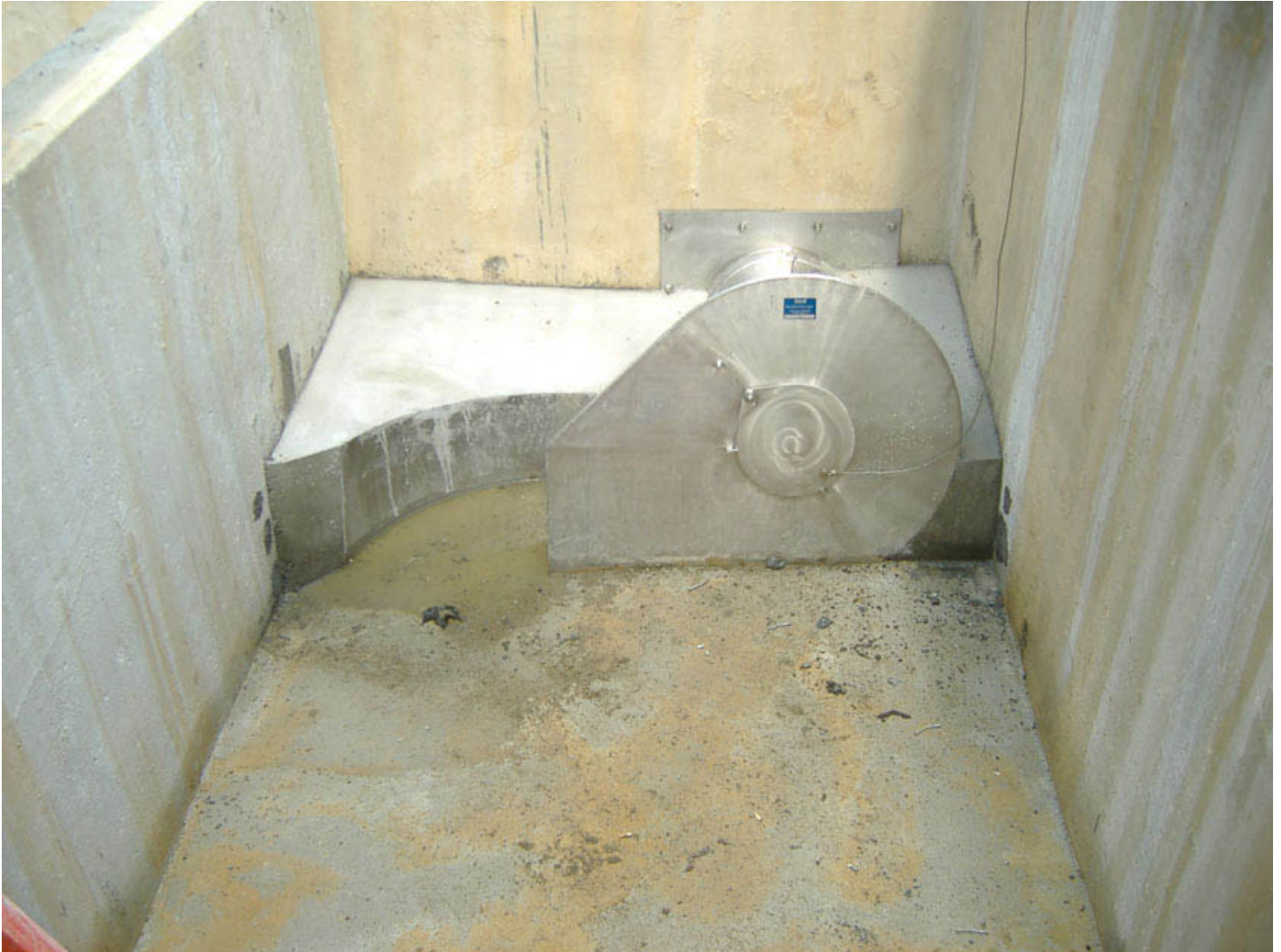
An example of a low flow device in Philadelphia
