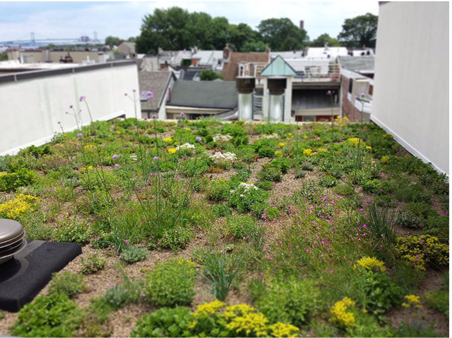
An example of a green roof in Philadelphia
