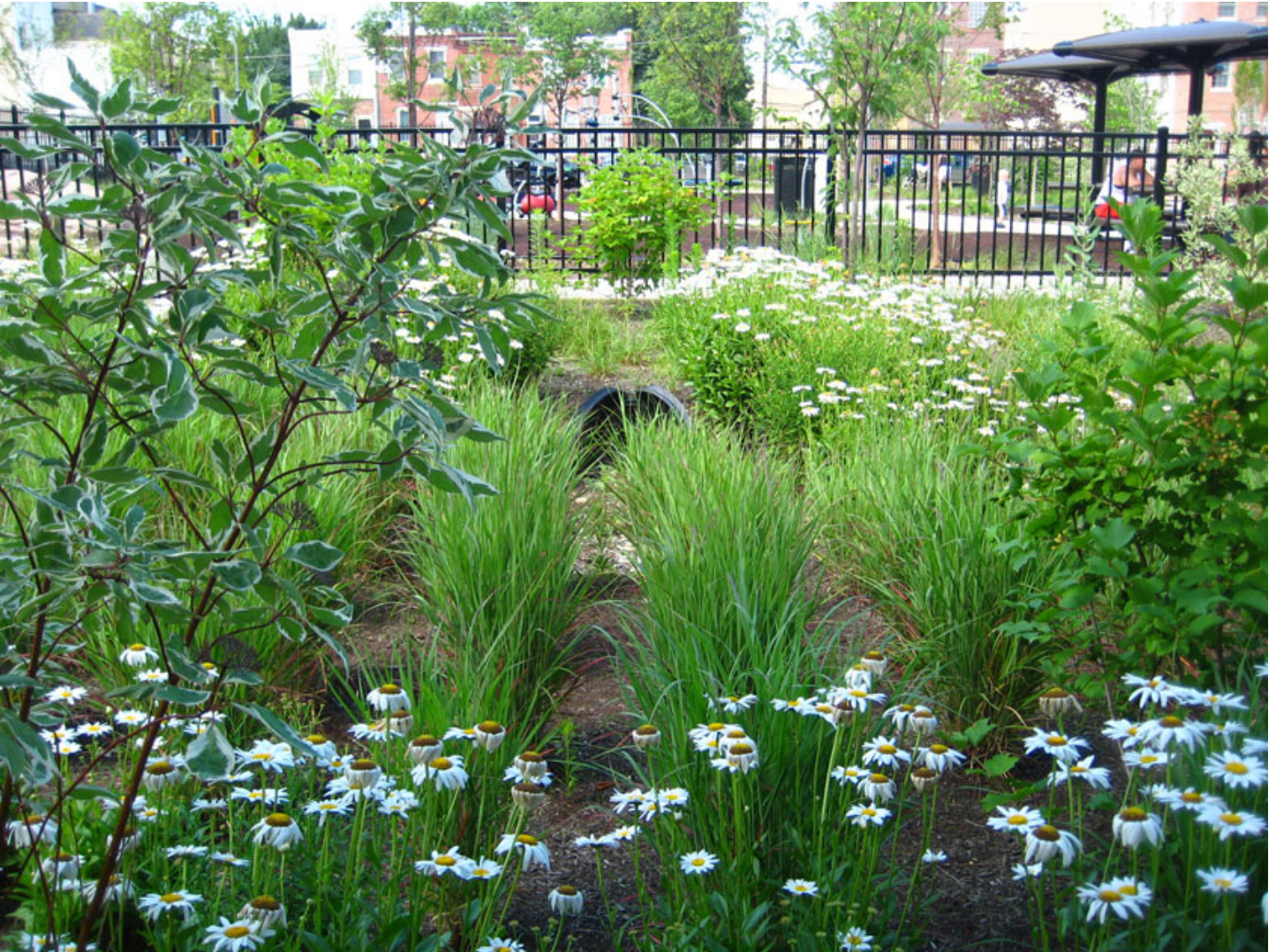
A bioinfiltration basin represents the Philadelphia Water Department's most preferred SMP.
