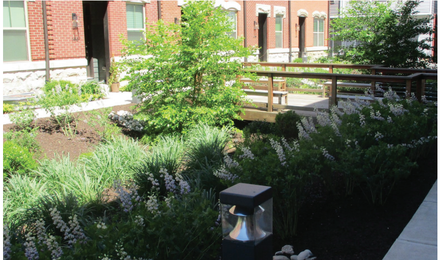
Installing a bioretention basin abutting existing impervious area can be an excellent Stormwater Management Banking and Trading strategy.
