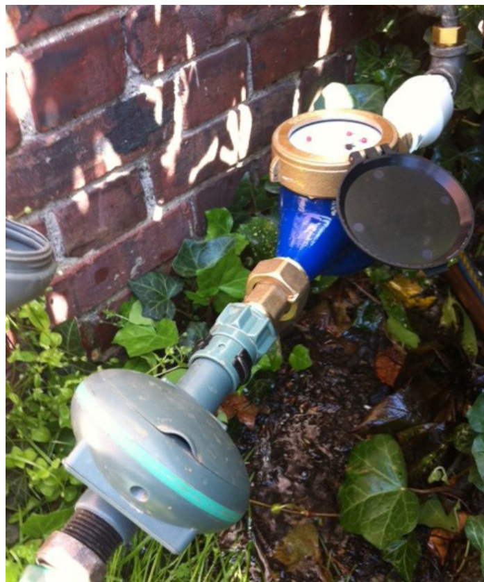
Example of a sub-meter installed on a water service adjacent to the garden.
