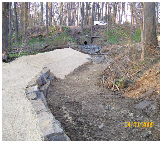
Figure 3-103: WSout513 conveyance channel during (left) and after (right) construction
