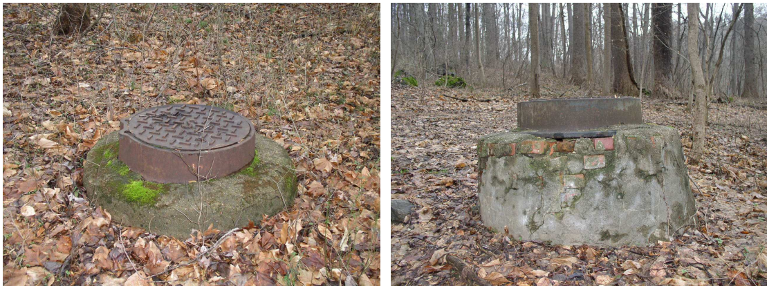
Figure 2-11: Examples of manholes assessed in infrastructure trackdown.
