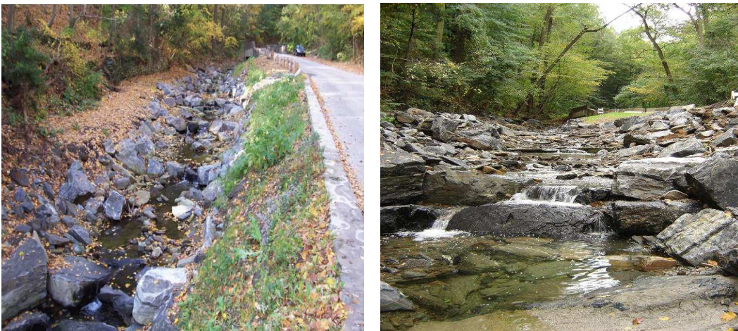
Figure 3-102: View of boulder step-pool system looking upstream (left): scour pool at the base of the step-pool system (right).
