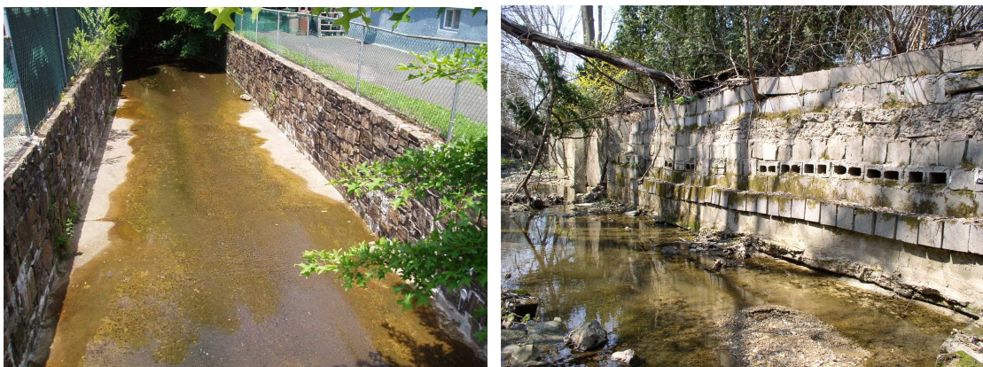
Figure 2-14: Examples of channels assessed in infrastructure trackdown.
