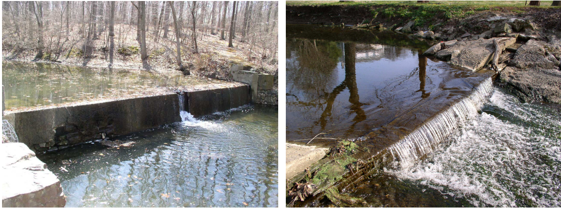
Figure 2-13: Examples of dams assessed in infrastructure trackdown.
