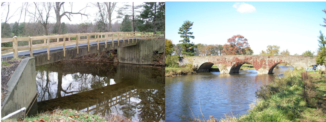
Figure 2-10: Examples of bridges assessed in infrastructure trackdown
