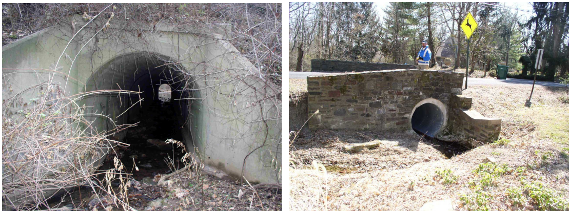
Figure 2-12: Examples of culverts assessed in infrastructure trackdown.
