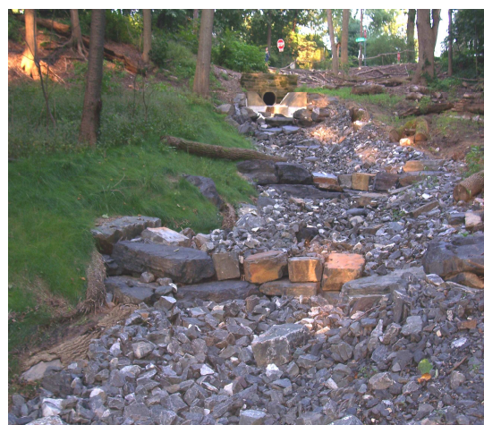
Figure 3-103: WSout513 conveyance channel during (left) and after (right) construction
