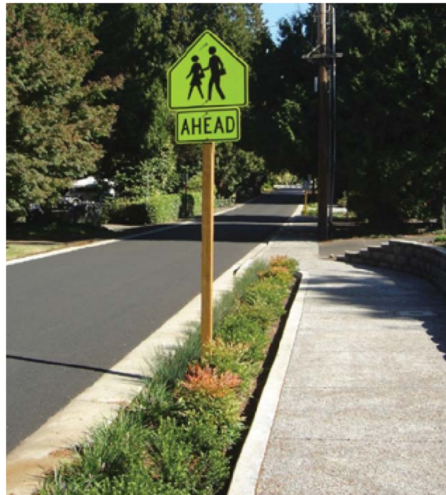
Figure 1-28. Example of a Green Gutter in Portland, Oregon (Image credit: PWD Green Streets Design Manual, 2014)
