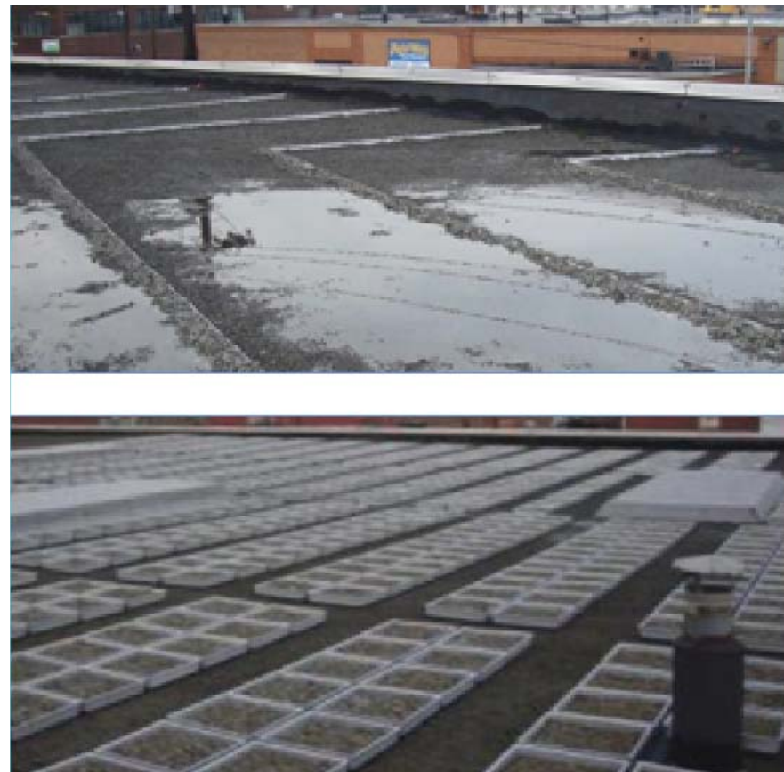
Figure 1-26. Examples of Blue Roofs in New York City (Image credit: 2012 NYC Green Infrastructure Pilot Monitoring Report)
