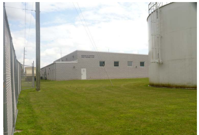
Borough of Kutztown Water Treatment Plant
