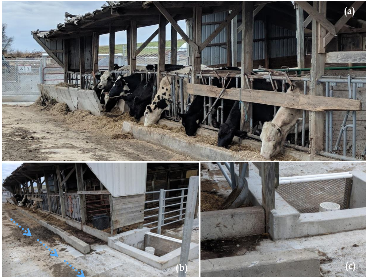
Figure 5-3: Youse Farm (a) Pitched Feeding Area (b) Stormwater Drainage collection at the corner of the barn (c) Drain to Collect Stormwater Runoff with Screen to Capture Large Debris
