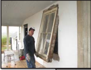
Exterior Window Repair
