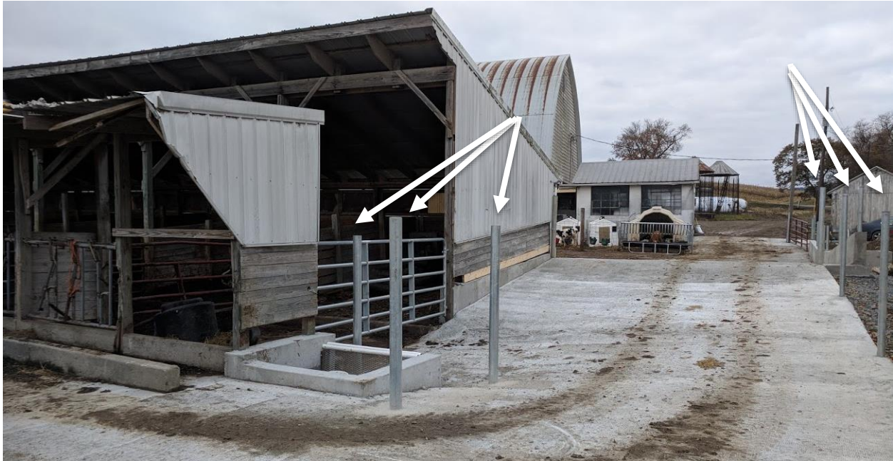
Figure 5-4: Youse Farm – Fencing Posts and Heavy Use Area
