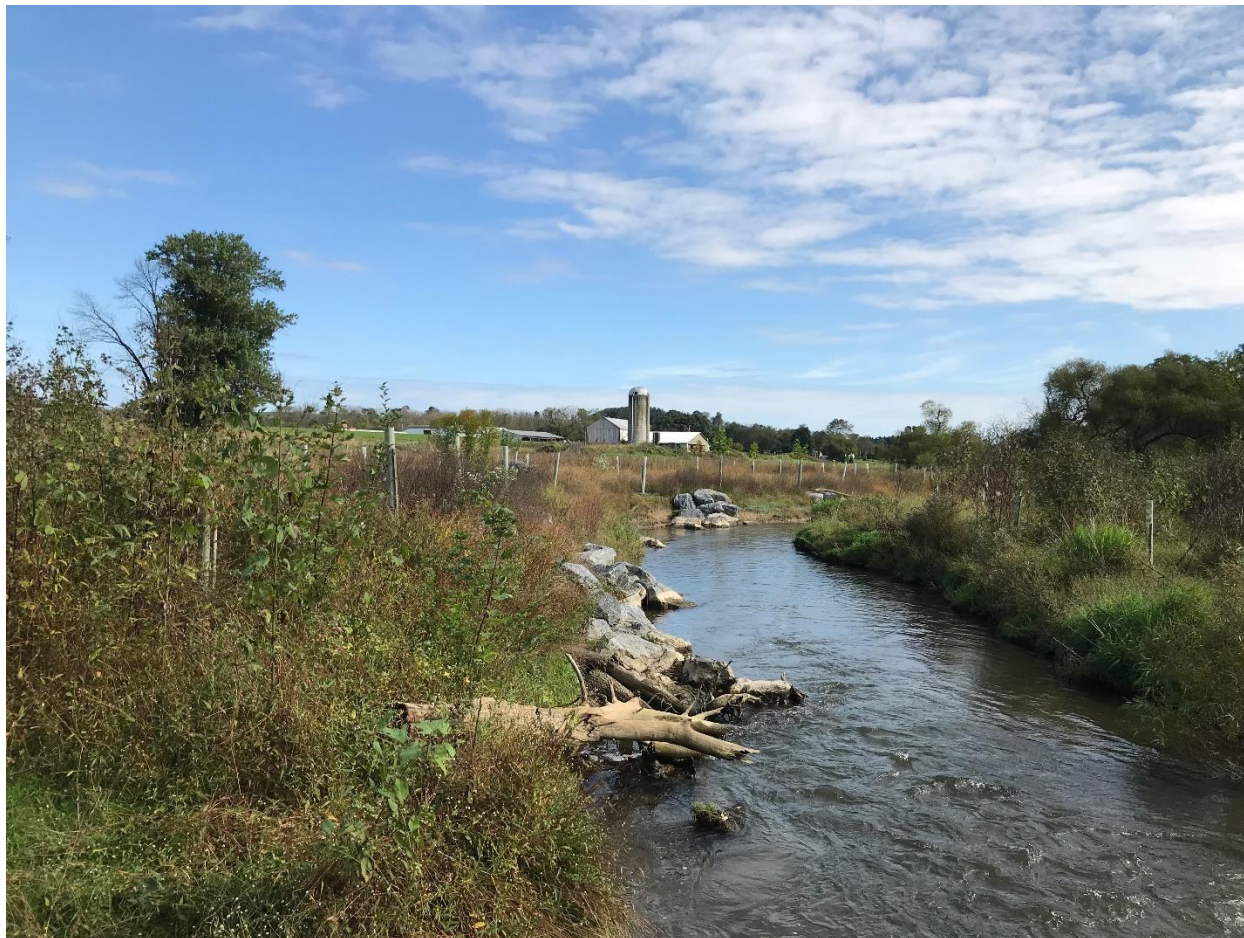
Figure 4-22: Irish Creek Project (October 2018) - Barbs Installed to Stabilize Left Bank
