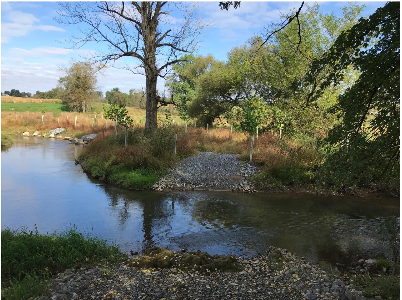
Figure 4-24: Irish Creek Project (October 2018) Stream Crossing
