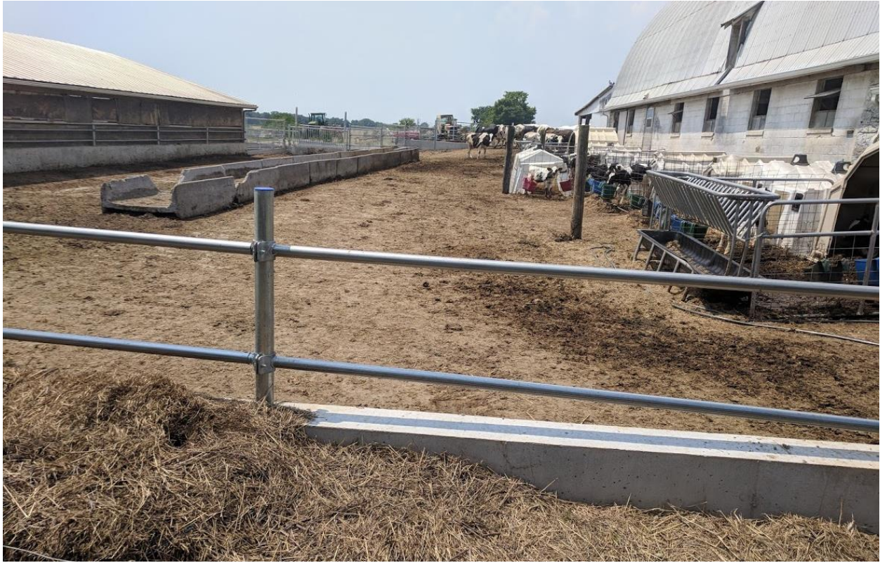
Figure 4-18: Youse Farm Cemented Heavy Use Area (June 2018)
