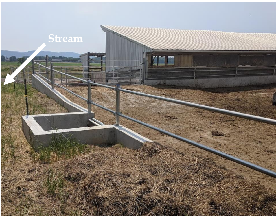
Figure 4-19: Youse Farm Cemented Heavy Use Area with Exclusion Fencing and Stormwater Runoff Collection Drain (June 2018)
