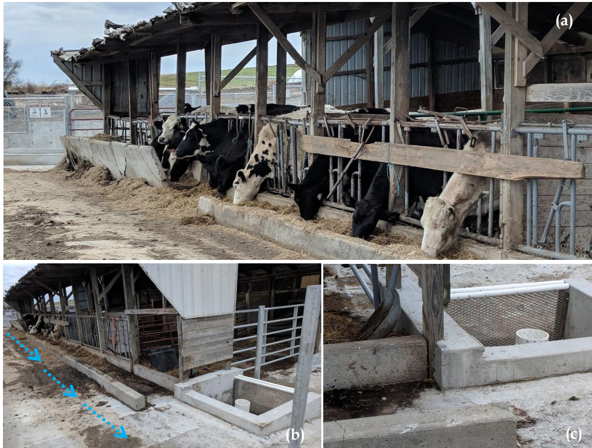
Figure 4-17: Youse Farm (a) Pitched Feeding Area (b) Stormwater Drainage collection at the corner of the barn (c) Drain to Collect Stormwater Runoff with Screen to Capture Large Debris
