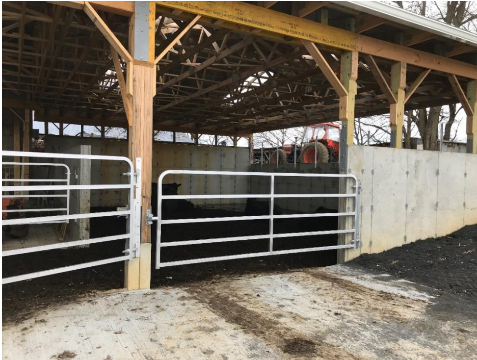
Figure 4-12: Cement Dry-Roofed Manure Storage Area at A. Burkholder Farm (November 2018)
