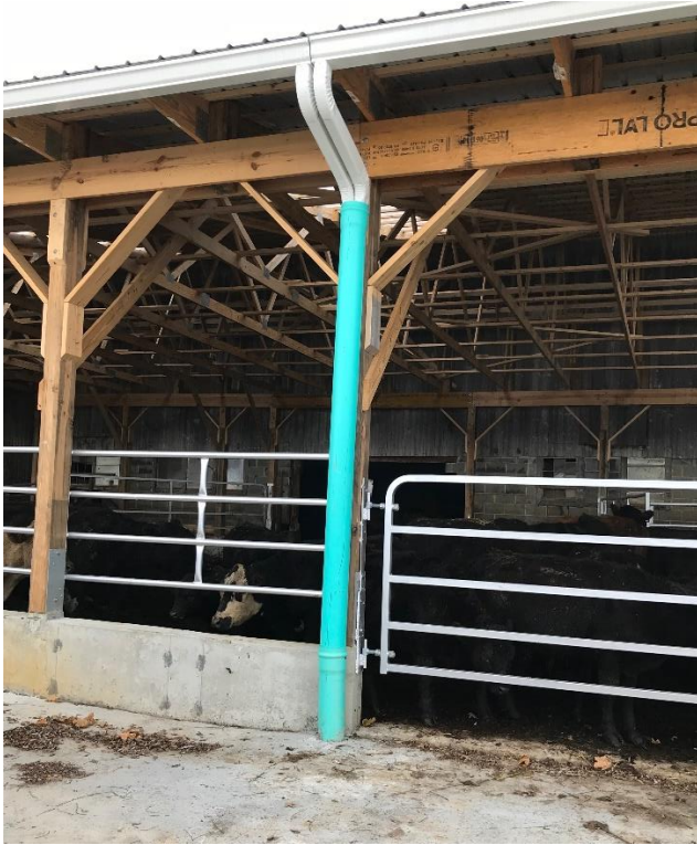
Figure 4-13: Manure Storage Area Rain Gutters at A. Burkholder Farm (November 2018)
