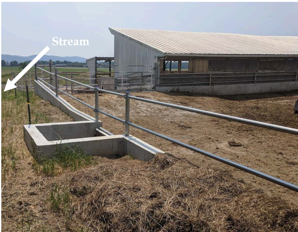
Figure 4-23: Youse Farm Cemented Heavy Use Area with Exclusion Fencing and Stormwater Runoff Collection Drain (June 2018)
