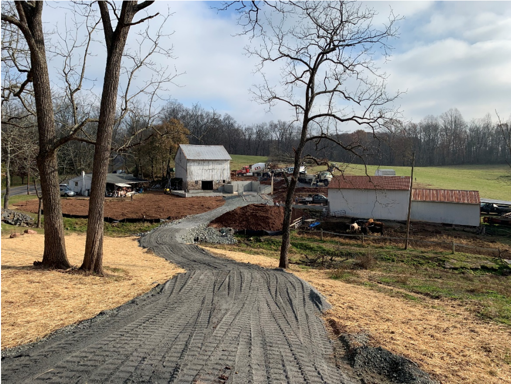
Figure 4-13: Love Farm During BMP Construction (Fall 2019)
