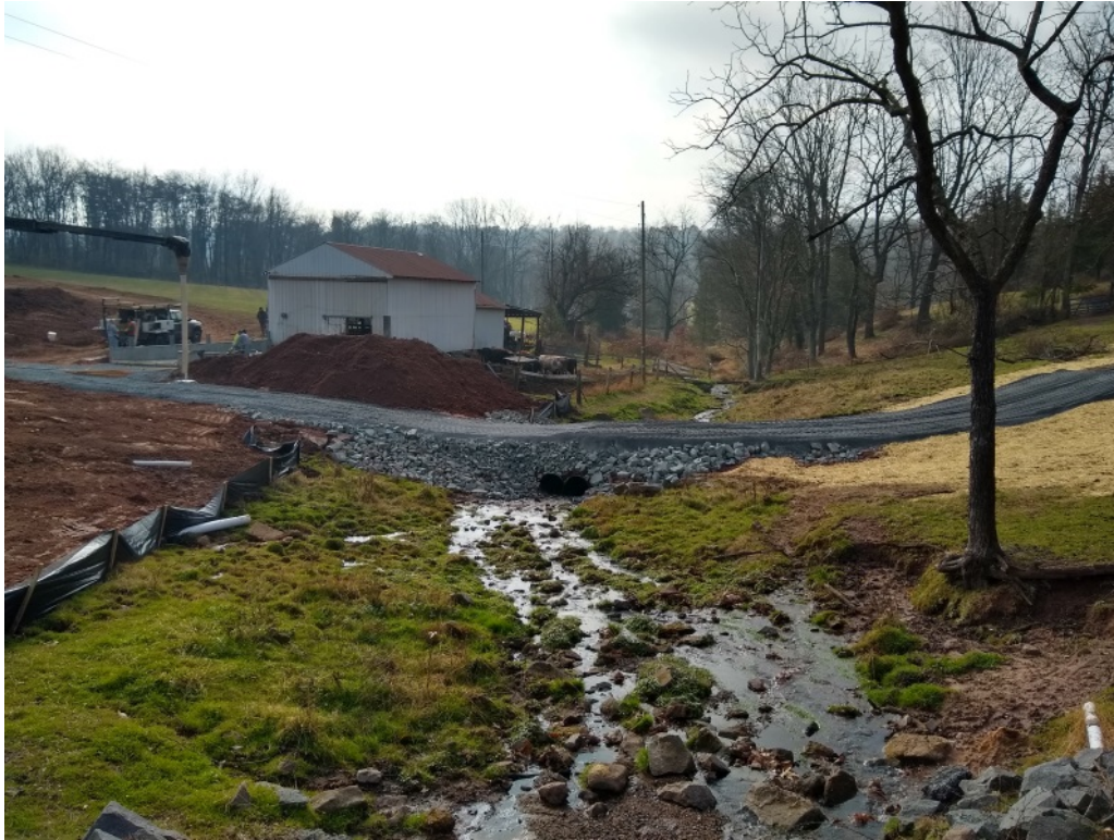
Figure 4-15: Protected Stream Crossing during BMP Construction (Fall 2019)
