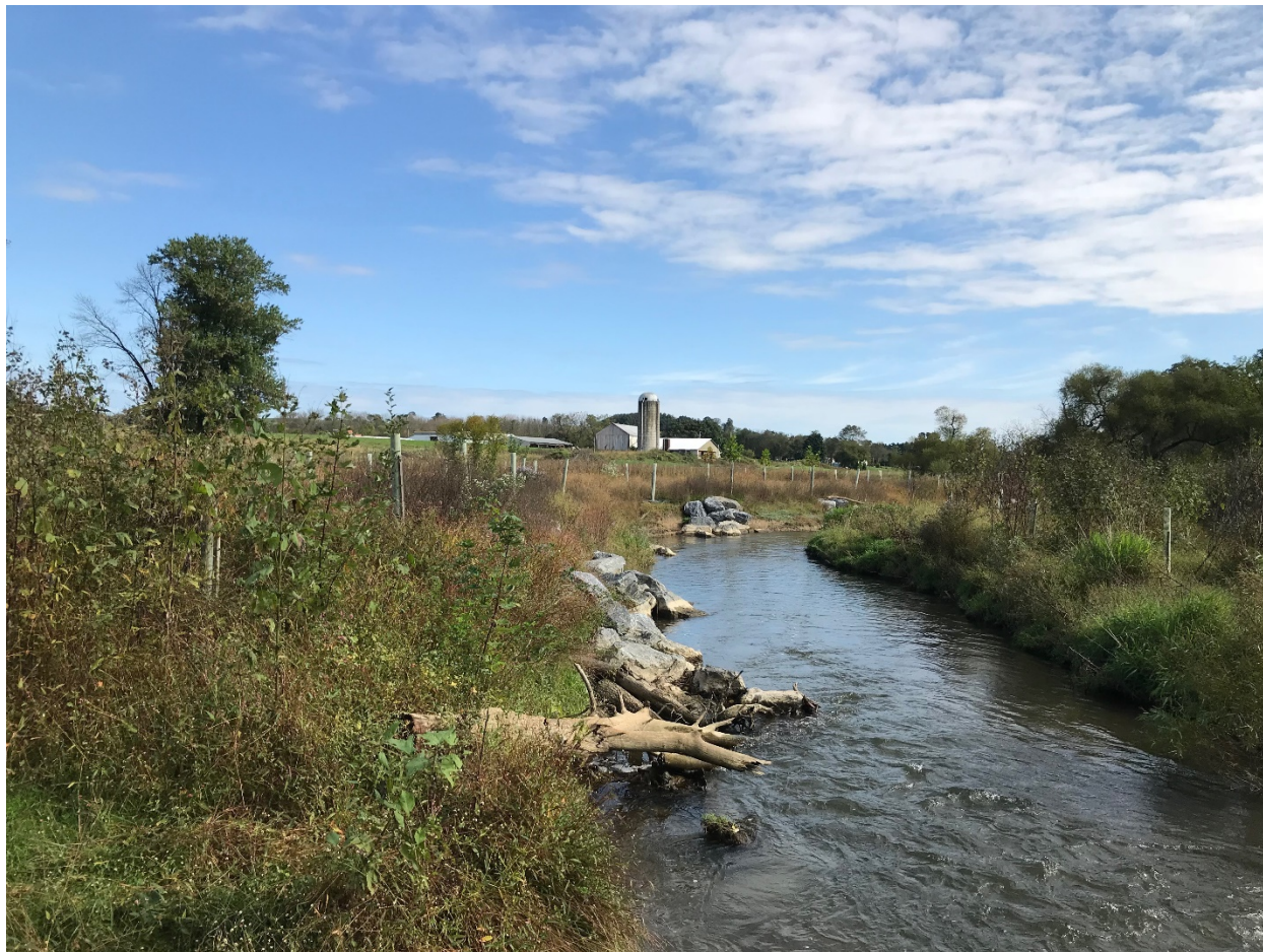
Figure 4-26: Irish Creek Project (October 2018) - Barbs Installed to Stabilize Left Bank
