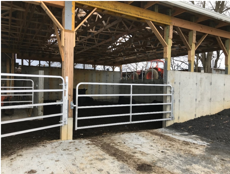
Figure 4-16: Cement Dry-Roofed Manure Storage Area at A. Burkholder Farm (November 2018)
