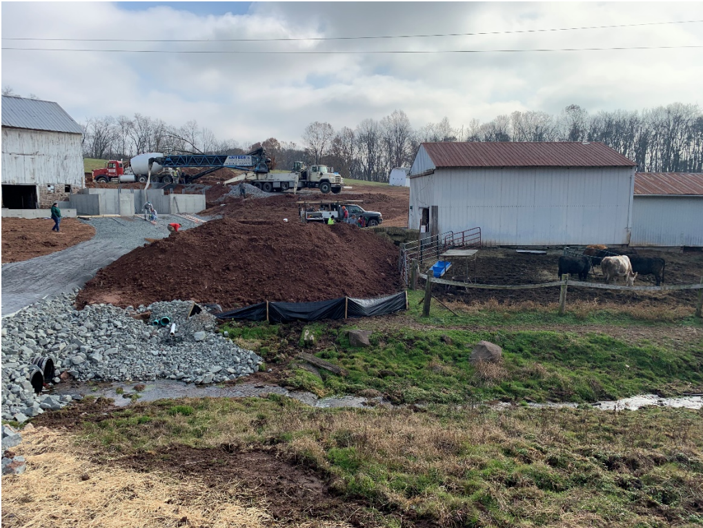
Figure 4-14: Construction of Roofed Stackpad and Erosion Control Measures (Fall 2019)
