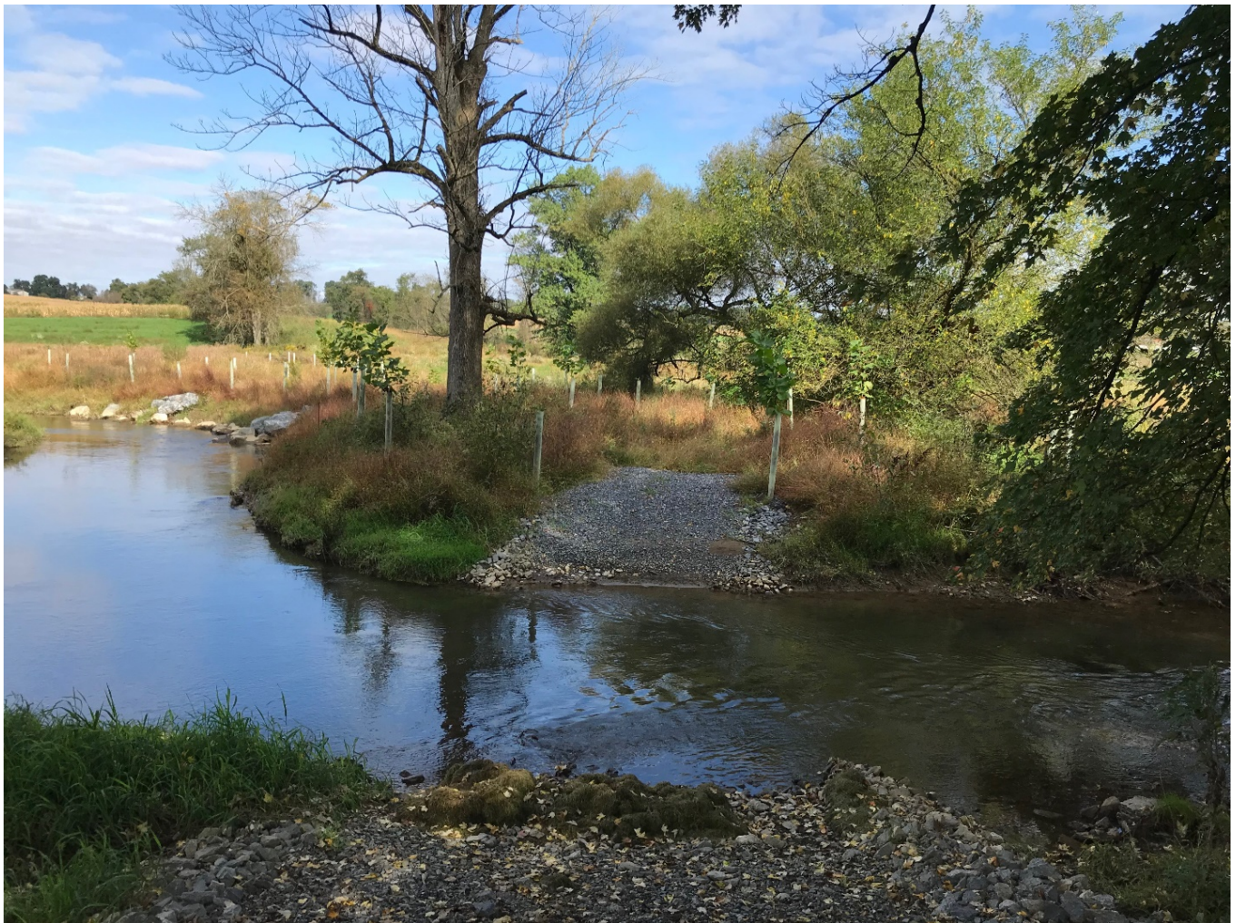
Figure 4-28: Irish Creek Project (October 2018) Stream Crossing
