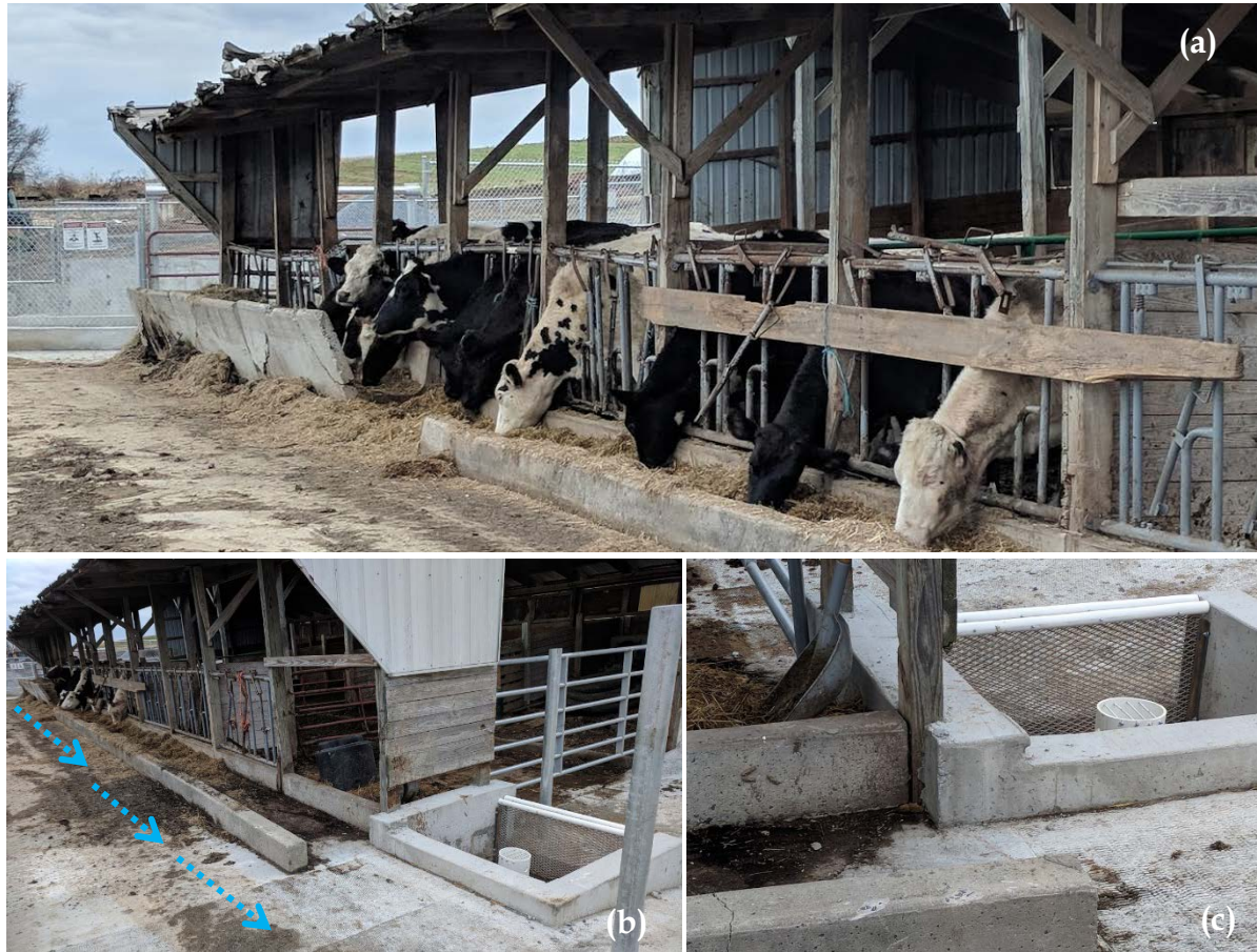
Figure 4-21: Youse Farm (a) Pitched Feeding Area (b) Stormwater Drainage collection at the corner of the barn (c) Drain to Collect Stormwater Runoff with Screen to Capture Large Debris
