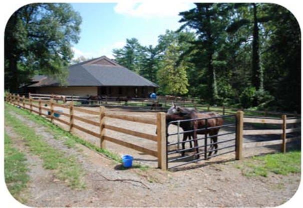
Post Construction Heavy Use Area 2
