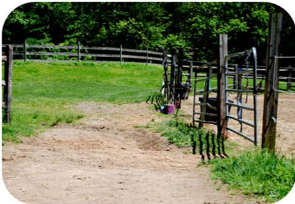
Pre-Construction Heavy Use Area 3
