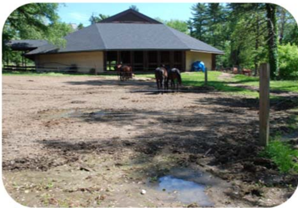
Pre-Construction Heavy Use Area 2
