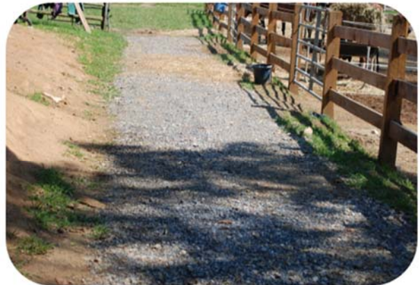
Post Construction Heavy Use Area 3
