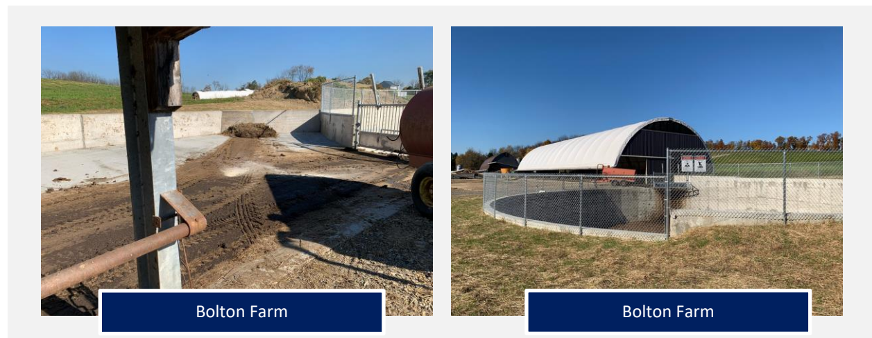
Figure 4-10: Bolton Farm paved manure transfer area (left) and 6-month capacity liquid manure storage basin (right) Photo Credit: PWD 2021
