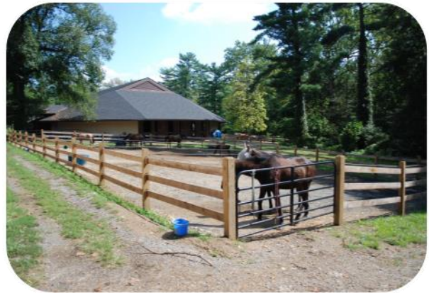
Post Construction Heavy Use Area 2
