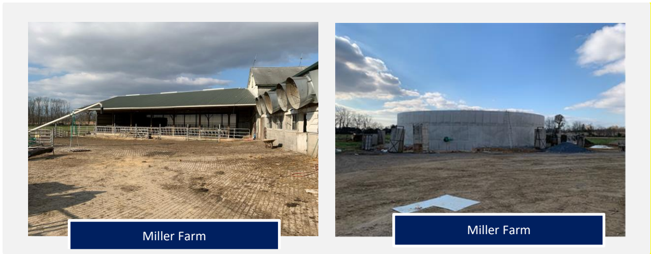
Figure 4-11: Miller Farm paved reception area with manure storage pit and pumping system (left) and six-month liquid manure storage basin (right). Photo Credit: PWD 2021
