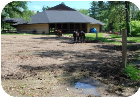
Pre-Construction Heavy Use Area 2
