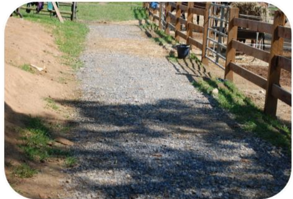
Post Construction Heavy Use Area 3
