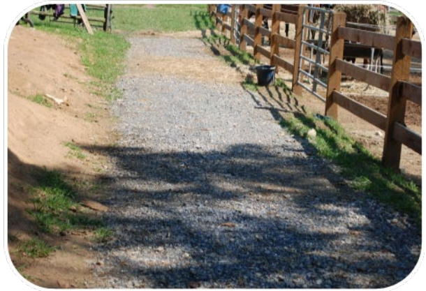
Post Construction Heavy Use Area 3
