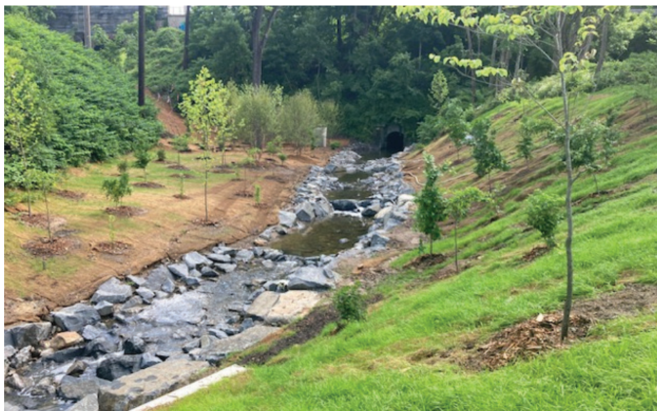
Image showing landscaping during construction along Cresheim Creek
