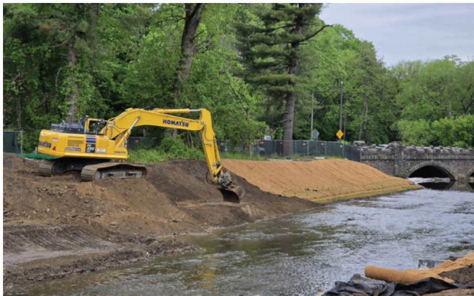
Image showing stream bank grading during construction along Cobbs Creek
