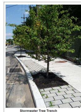
Stormwater Tree Trench
