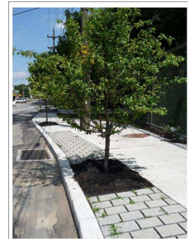
Stormwater Tree Trench
