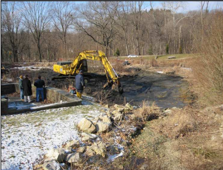
Dredging of forebay pond. View from footbridge.
