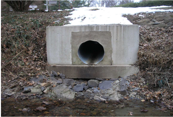
Figure 2-9: Example of an outfall point assessed in infrastructure trackdown
