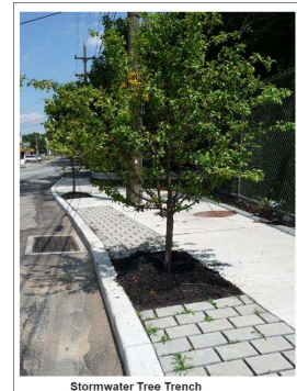
Stormwater Tree Trench
