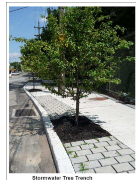
Stormwater Tree Trench
