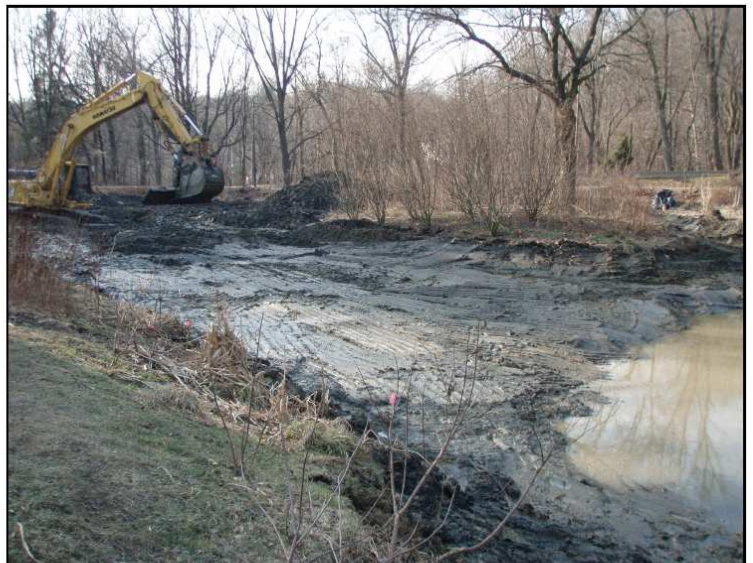
Grading the southwest area away from forebay pond.
