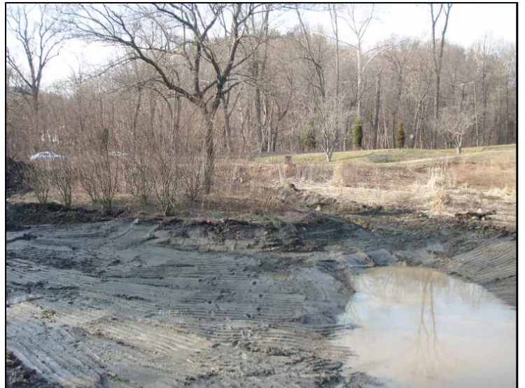
Grading around forebay pond area.
