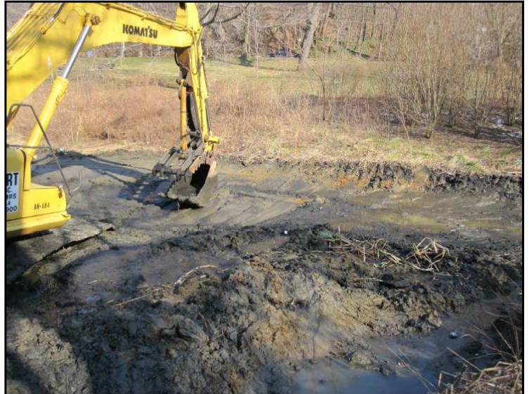
Dredging of forebay pond.
