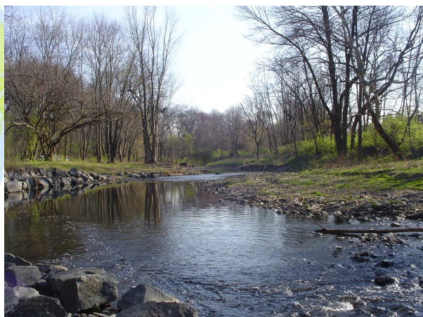
Downstream view of Cobbs Creek post construction
