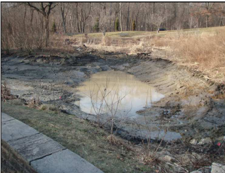
Forebay pond after dredging.
