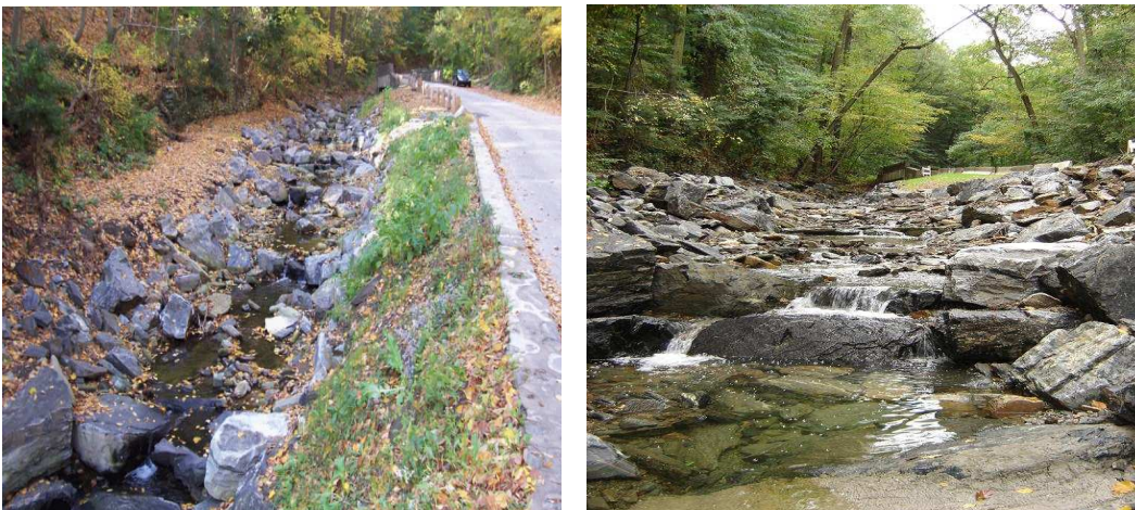
Figure 3-102: View of boulder step-pool system looking upstream (left): scour pool at the base of the step-pool system (right).
