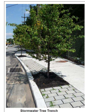
Stormwater Tree Trench
