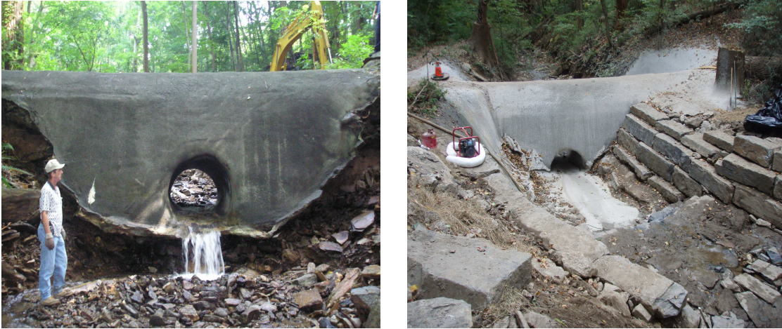
Figure 3-101: Upstream view of WScul116 pre-construction (left); Downstream view of WScul116 post-construction (right).
