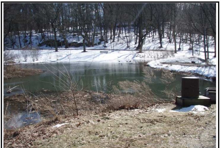
View from the outlet structure to Rittenhouse
