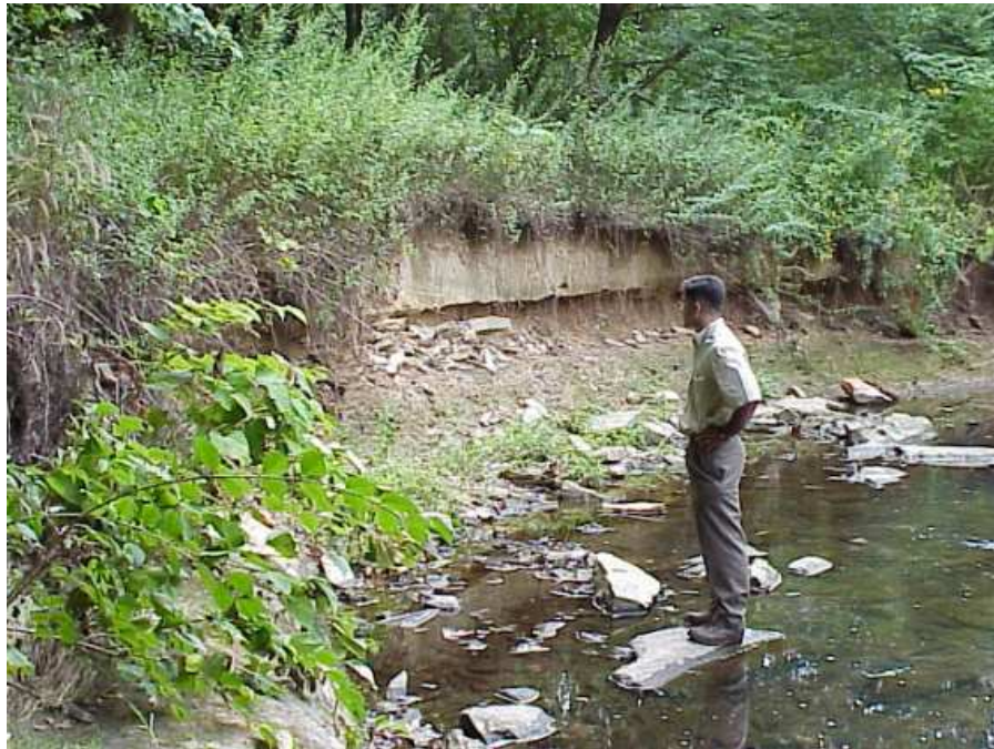
Photo 2 - Severe Bank Erosion along the Marshall Road Project Reach
