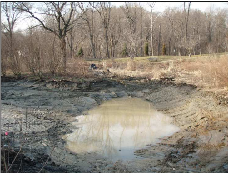
Dredged forebay pond. View from channel.
