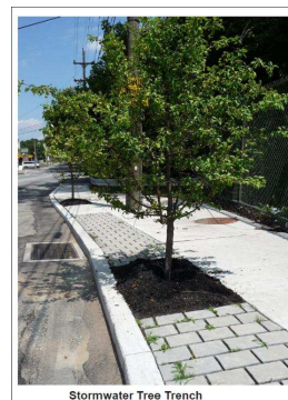
Stormwater Tree Trench
