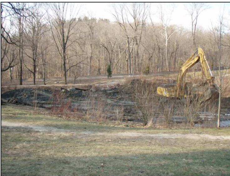
Dredging and grading southwest area.
