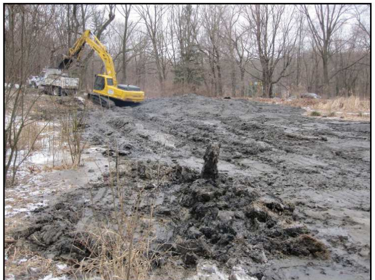
Loading dredged material onto trucks for transfer and disposal.
