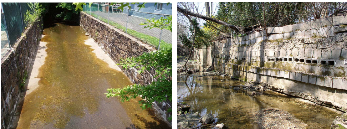
Figure 2-14: Examples of channels assessed in infrastructure trackdown.
