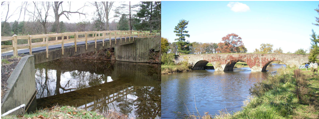
Figure 2-10: Examples of bridges assessed in infrastructure trackdown
