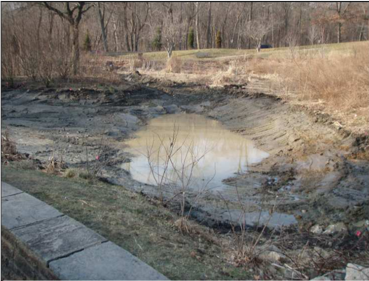
Dredged forebay pond. View from fountain.
