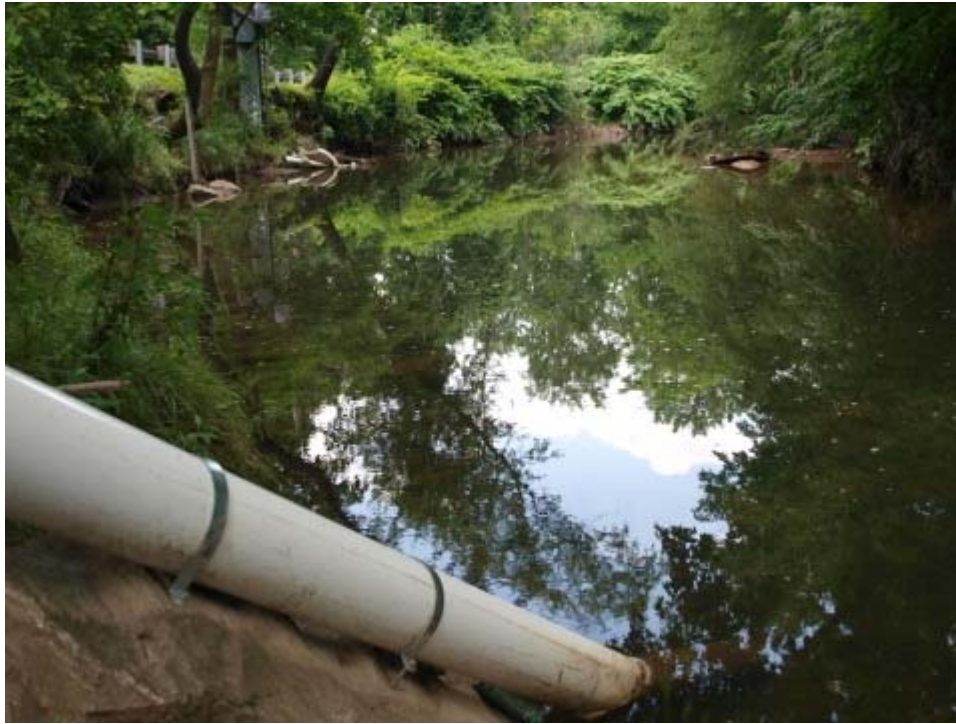
Figure 41. Gage 01465798, Poquessing Creek at Grant Ave., looking upstream
