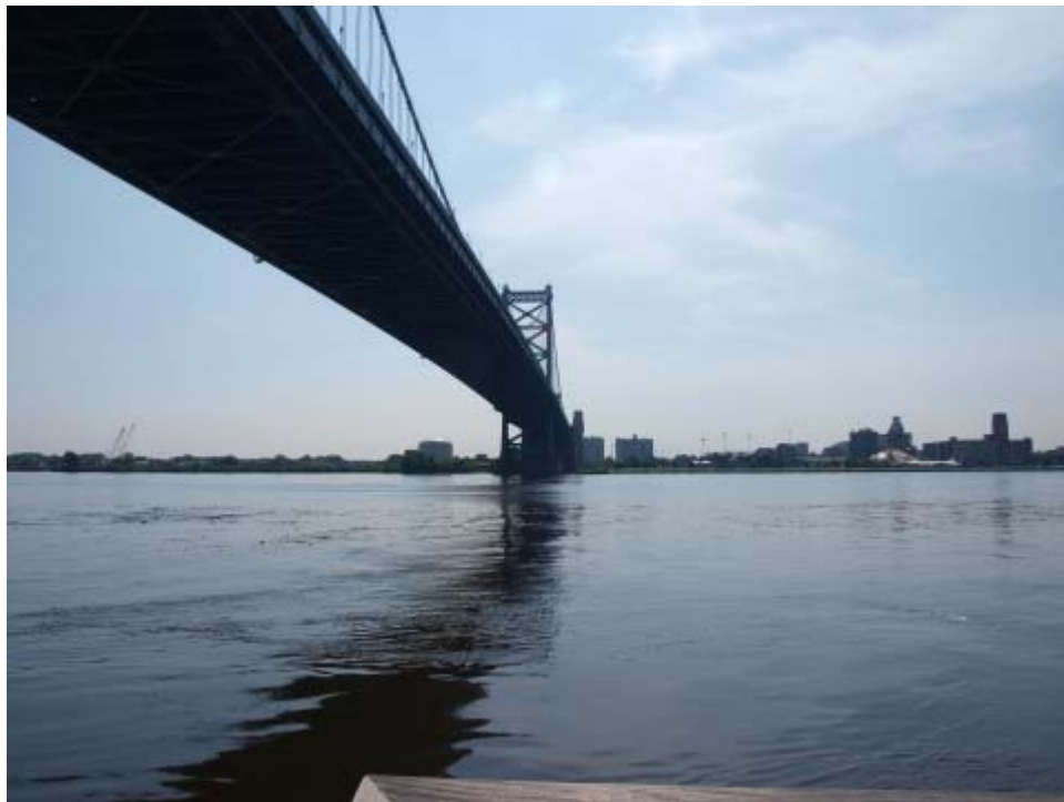
Figure 44. Delaware River at Ben Franklin Bridge, near Gage 01467200
