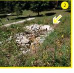
Stormwater Diversion Chamber #2 Outlet: Stormwater runoff from the Rittenhouse Avenue side of the Park is diverted into the Park as well. The outlet for this diversion chamber is also visible at the cascade. Refer to Site #1 for a description of the chamber \*Stream Daylighting
