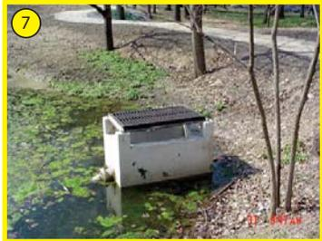
goes above 2 feet, it will spill into the outlet structure.
