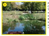
Permanent Pool (Pool #1), Channels, Collecting Pool (Pool #2) The permanent pool is located at the base of the cascade. It removes the majority of the fine particulate matter in the stormwater wetland. The collecting pool is a smaller version of the permanent pool. It is located directly across - on the other side of the wetland where the outlet structure is located. The surrounding channels reduce the velocity of the flow. Water Quality Sampling
