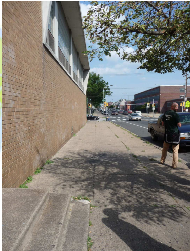
Sidewalk in front of Recreation Center
