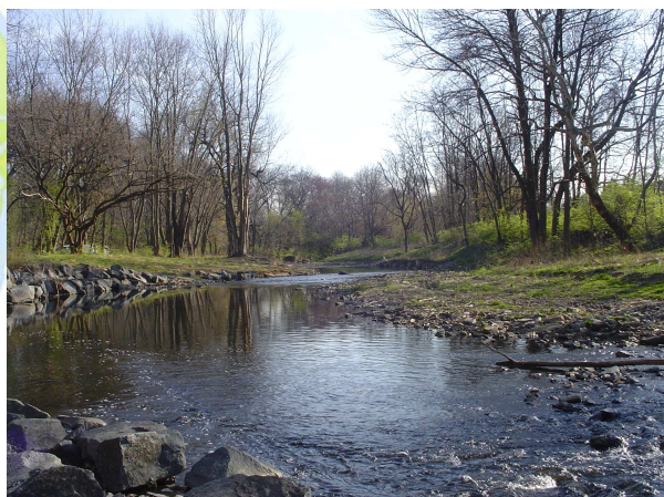
Downstream view of Cobbs Creek post construction
