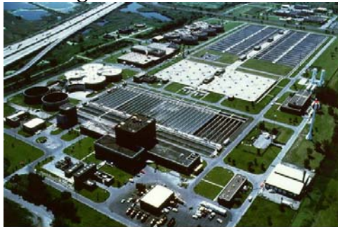
Figure 4-25 Municipal Wastewater Treatment Plant
