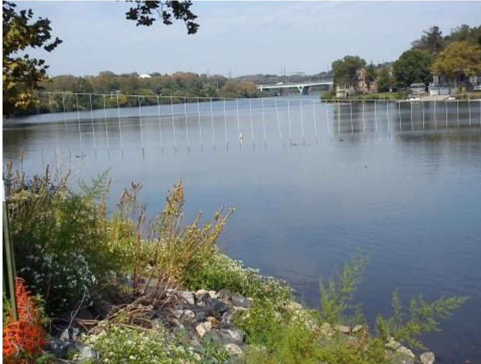
Figure 61. Gage 01474500, Schuylkill River at the Fairmount Dam, looking upstream
