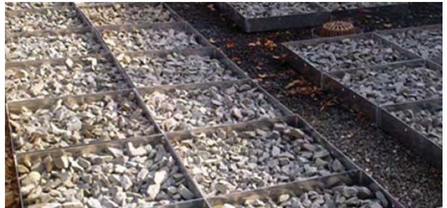
Figure 1-29. Examples of Blue Roofs in New York City (Image credit: Gowanus Canal Watershed, Hazen and Sawyer)
