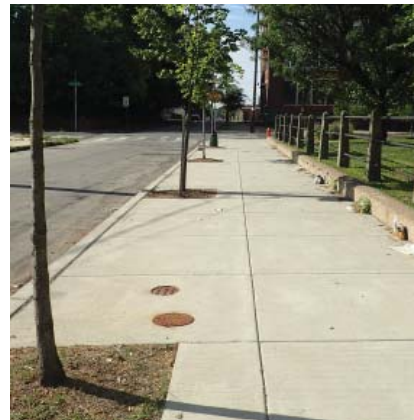
Figure 1-1. Examples of Stormwater Tree Trenches in Philadelphia
