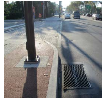
Figure 1-11. Examples of Infiltration/Storage Trenches in Philadelphia
