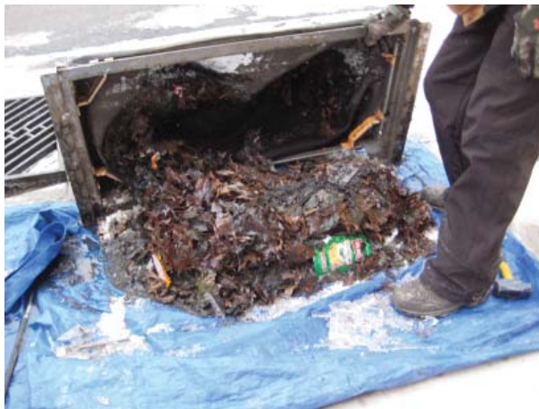
Figure 2-2. Cleaning of Pretreatment Device for a Highway Grate Inlet
