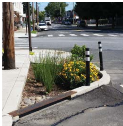
Figure 1-6. Examples of Stormwater Bump-outs in Philadelphia
