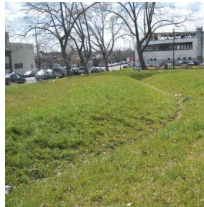
Figure 1-17. Examples of Stormwater Swales in Philadelphia
