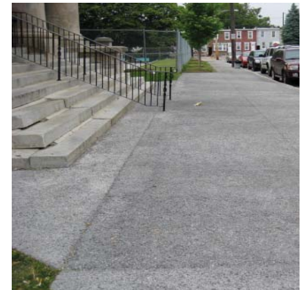
Figure 1-23. Examples of Pervious Pavement in Philadelphia
