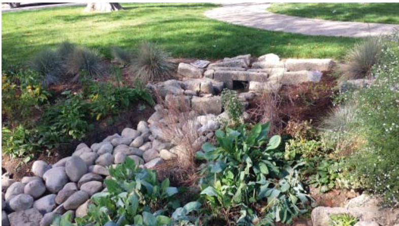
Figure 2-4. Extension of a Velocity Dissipator
