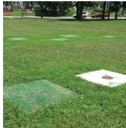
Figure 1-11. Examples of Infiltration/Storage Trenches in Philadelphia
