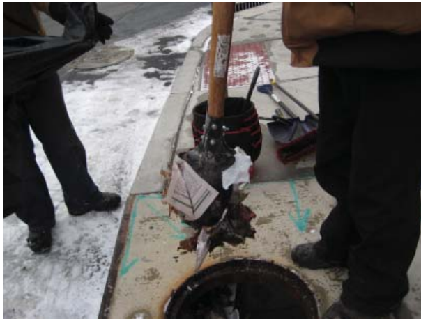
Figure 2-1. Cleaning of Pretreatment Device for a City Inlet
