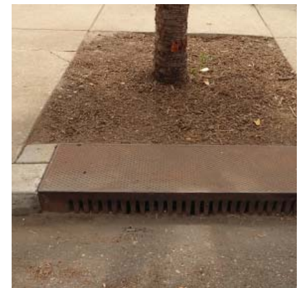
Figure 1-19. Examples of Stormwater Trees in Philadelphia
