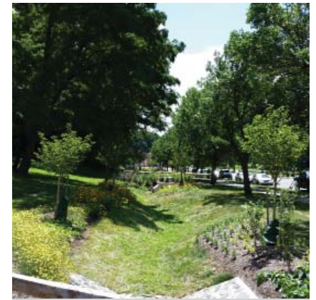
Figure 1-17. Examples of Stormwater Swales in Philadelphia
