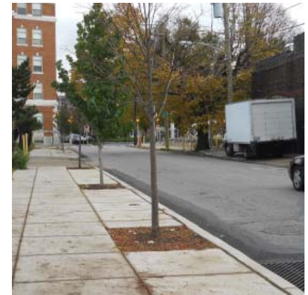
Figure 1-1. Examples of Stormwater Tree Trenches in Philadelphia
