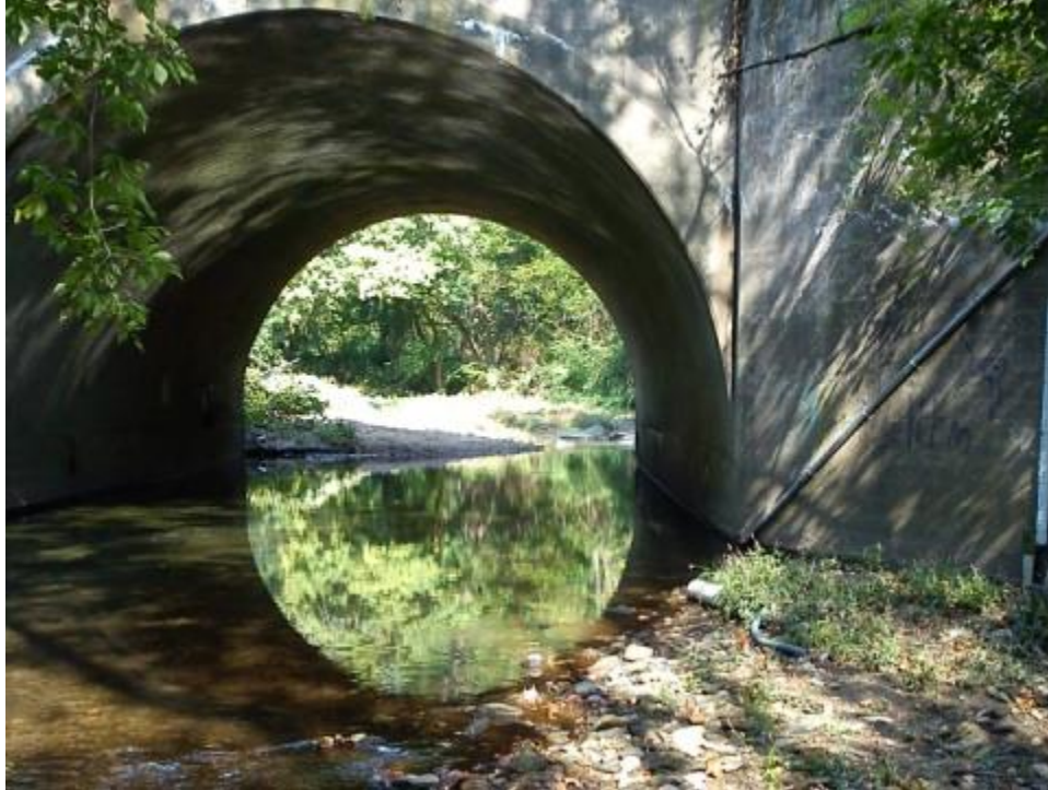
Figure 23. Gage 01475530, Cobbs Creek at Rte. 1, looking upstream
