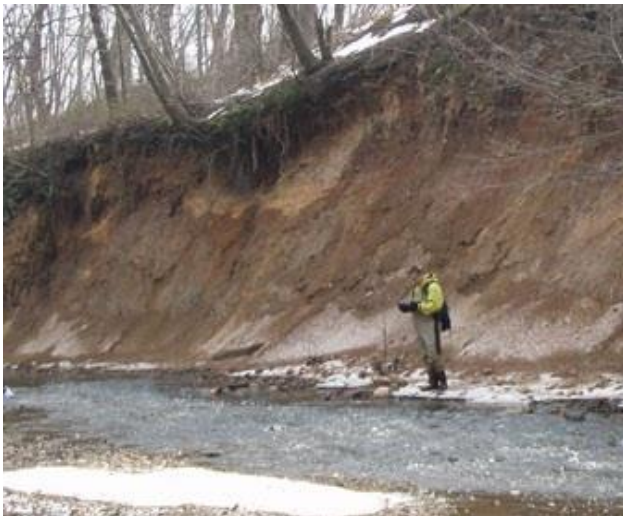
Figure 1. Eroded stream bank at Poquessing Creek
