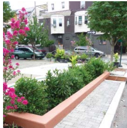
Figure 1-9. Examples of Stormwater Planters in Philadelphia
