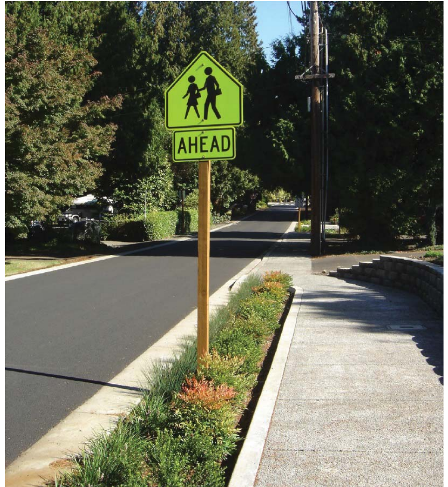
Figure 1-31. Example of a Green Gutter in Portland, Oregon (Image credit: PWD Green Streets Design Manual, 2014)
