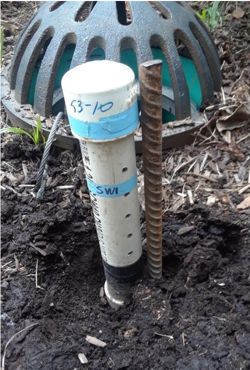
Figure 5-8 – Shallow Well & Rebar Alignment
