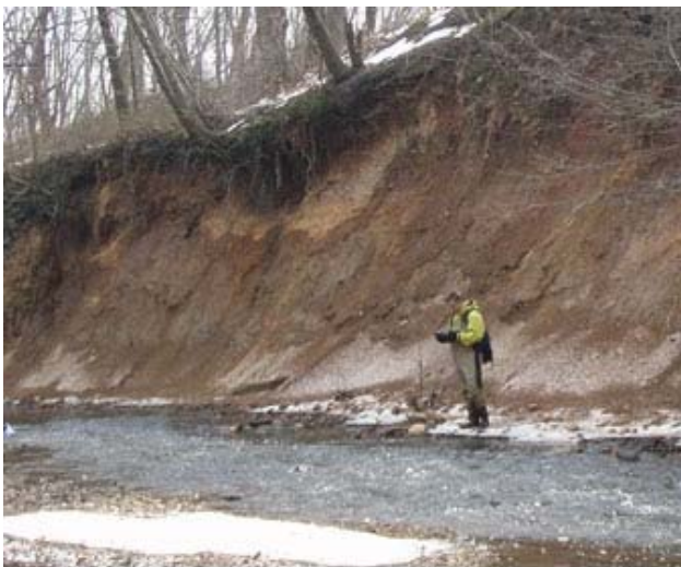
Figure 1. Eroded stream bank at Poquessing Creek
