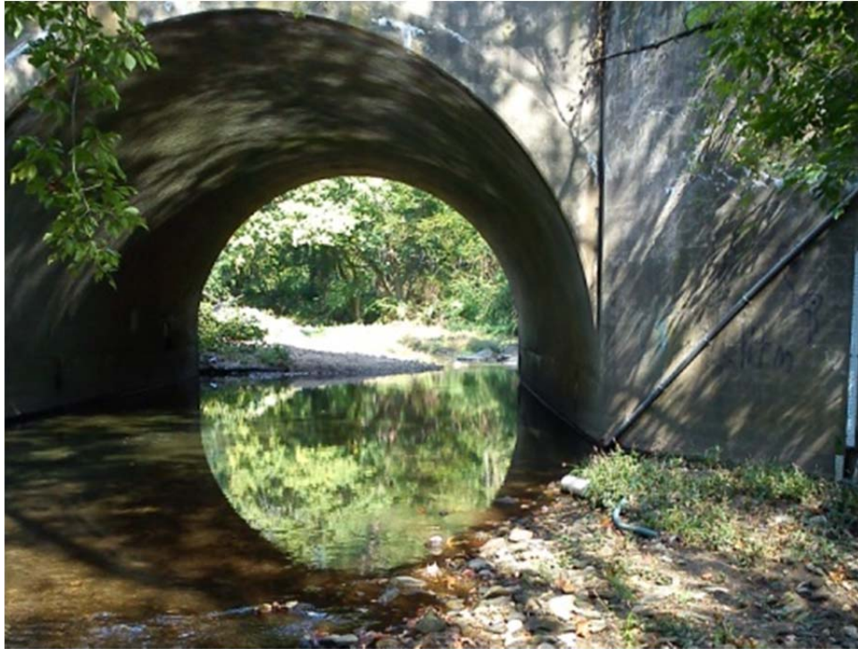
Figure 23. Gage 01475530, Cobbs Creek at Rte. 1, looking upstream
