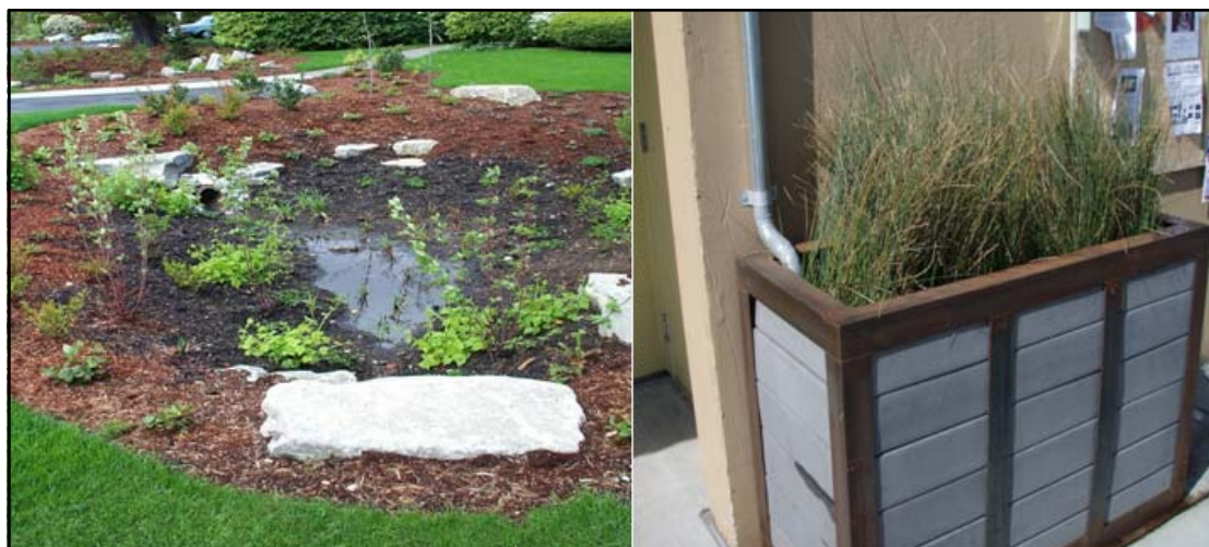
Figure 10-28 Examples of a Rain Garden and Disconnected Rain Spout for Residential Areas
