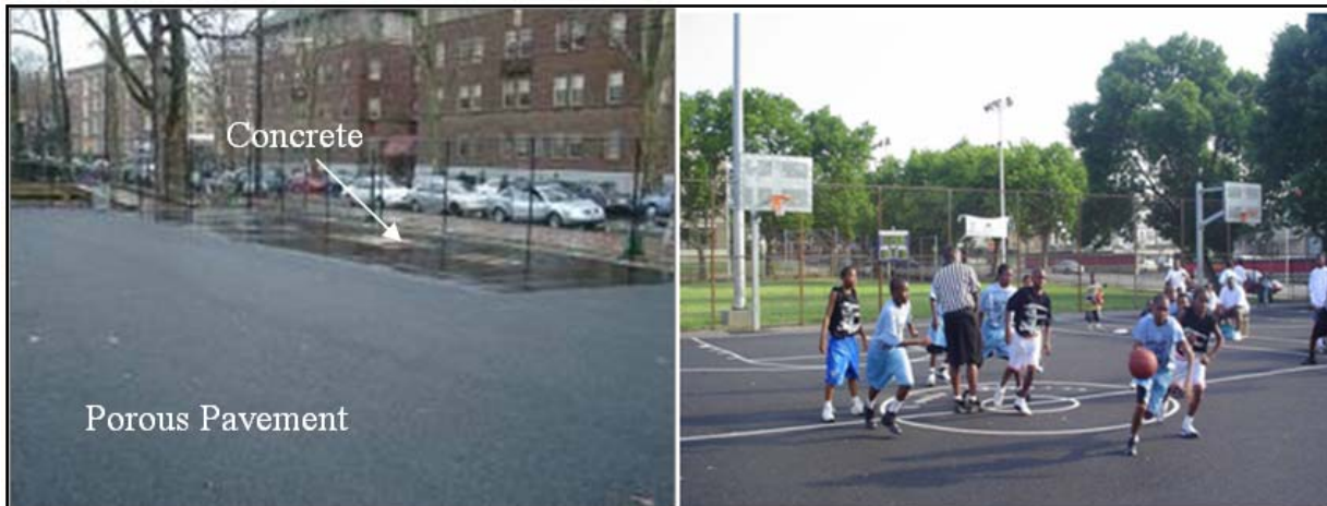
Figure 10-15 Porous Pavement Examples
