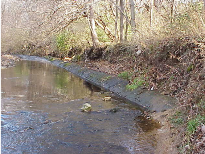
Figure 1-5 Marshall Road Pre-Restoration (Note Exposed Interceptor)
