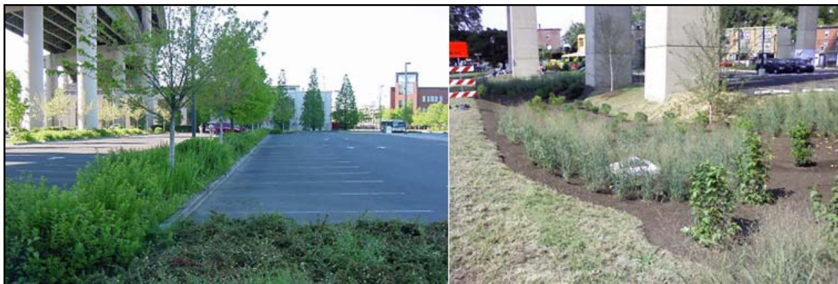
Figure 10-19 Examples of Green Retrofit Parking Projects
