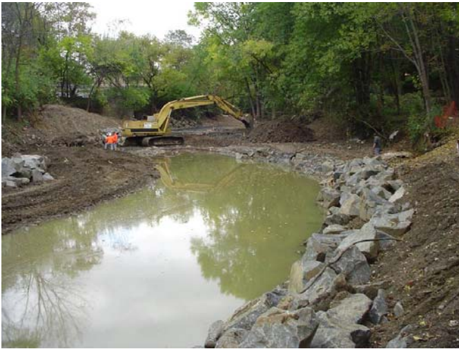
Figure 1-6 Marshall Road Under Construction – 2004
