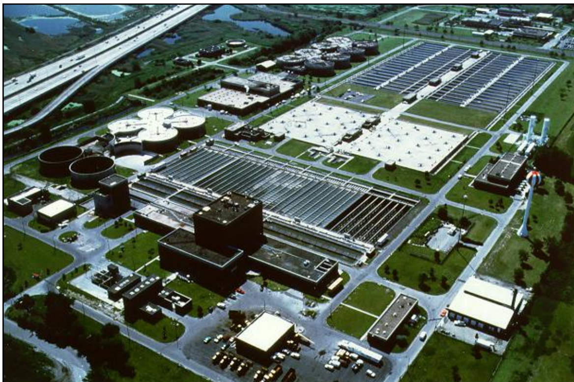
Figure 10-38 Image of PWD's Southwest Water Pollution Control Plant
