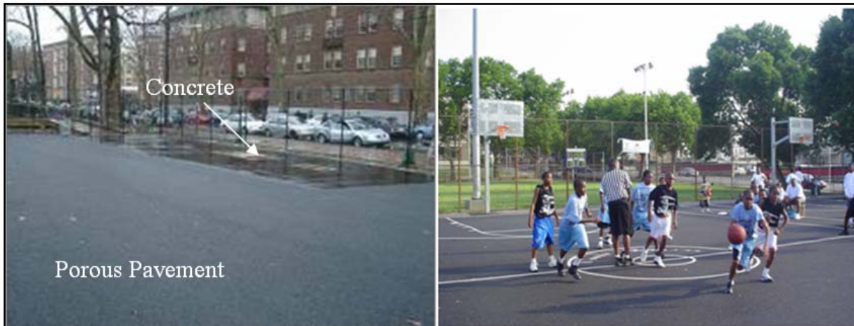
Figure 10-15 Porous Pavement Examples
