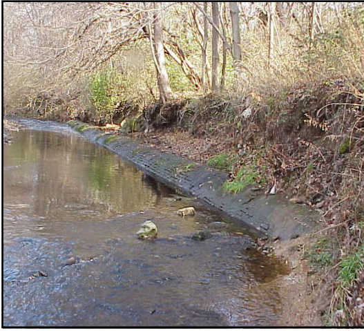
Figure 10-4 Before and After a Stream Restoration of Exposed Interceptor Pipe Along Marshall Road in the Cobbs Creek Watershed
