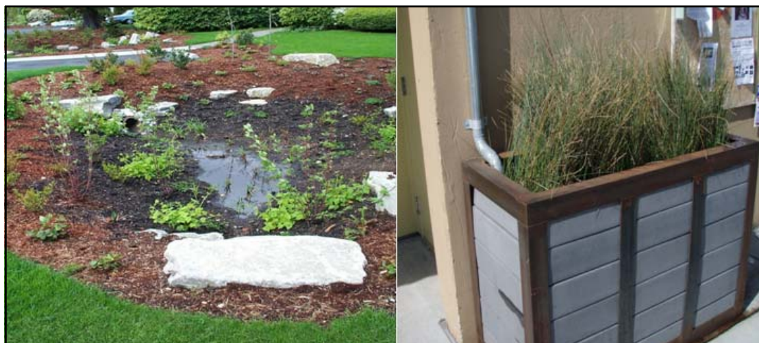
Figure 10-28 Examples of a Rain Garden and Disconnected Rain Spout for Residential Areas
