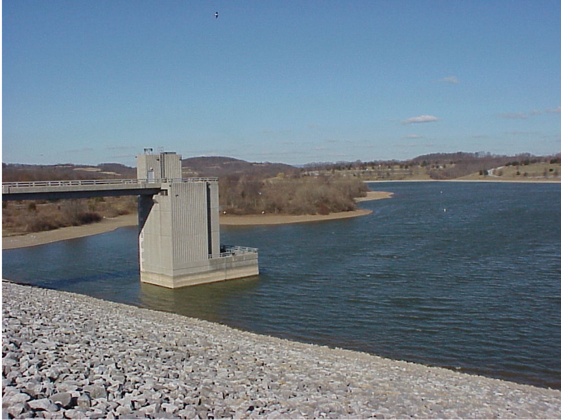
Blue Marsh Reservoir, Berks County, PA
