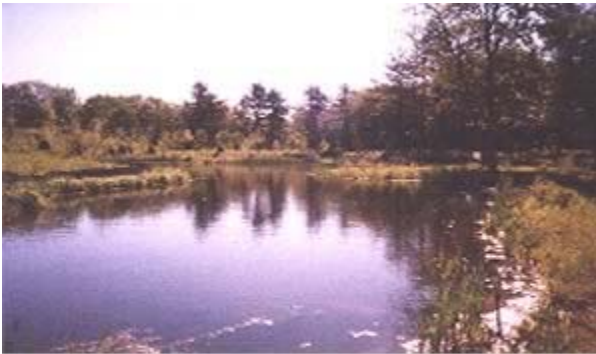
A storm water wetland detains storm water, removes pollutants, and provides habitat and aesthetic benefits (Source: The Bioengineering Group, Inc., no date)
