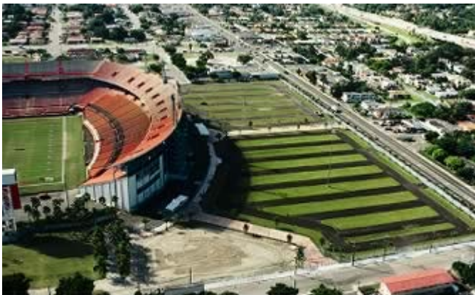
A green parking lot at the Orange Bowl in Miami, Florida (Source: Invisible Structures, no date)
