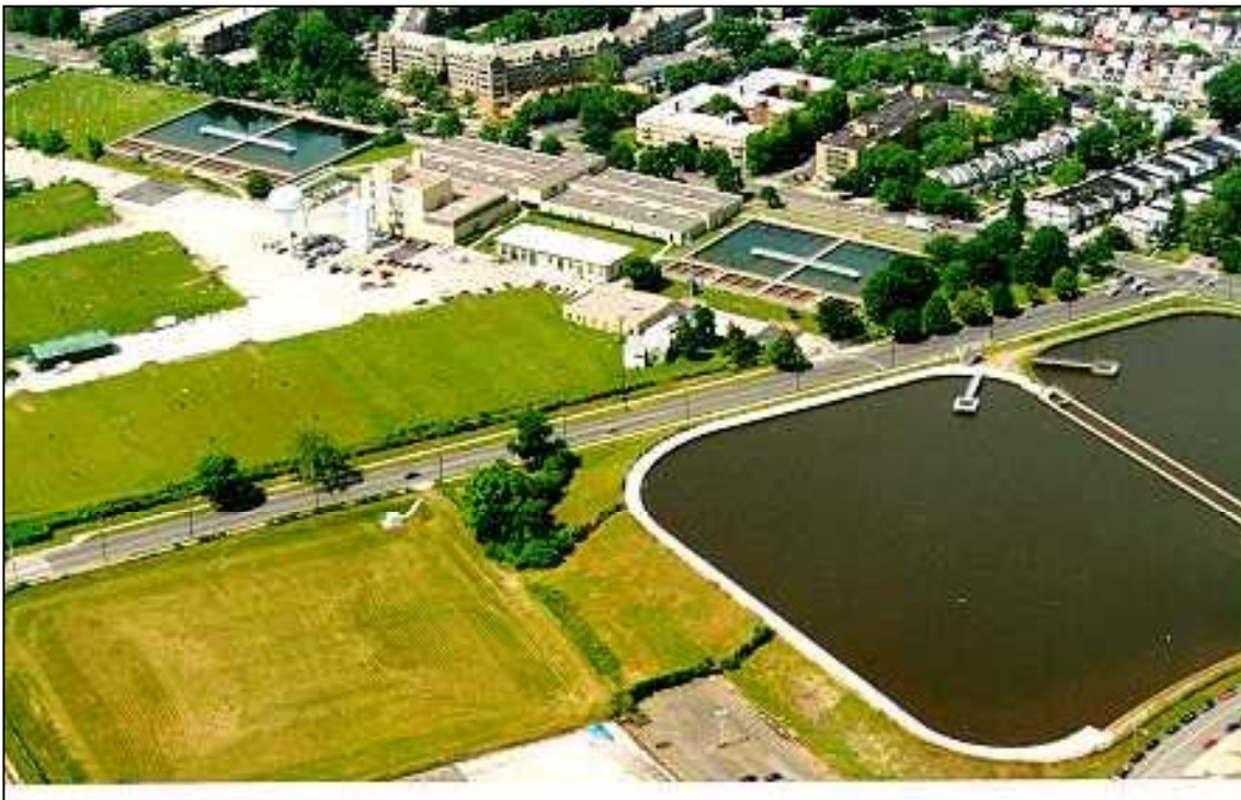
Figure 2.1.4-1 Philadelphia Water Department's Belmont Water Treatment Plant
