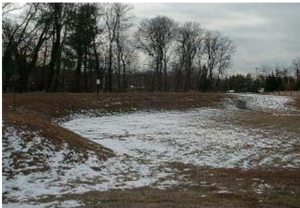
A dry extended detention pond is designed to temporarily detain runoff during storm events
