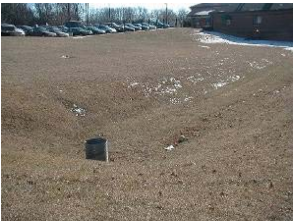
Infiltration basins are designed to collect storm water from impervious areas and provide pollutant removal benefits through detention and filtration
