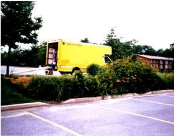
Bioretention areas can be used in parking areas to collect and treat storm water (Source: University of Maryland, 2000)
