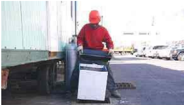
A worker inserts a catch basin insert for oil and grease, trash, debris, and sediment removal from storm water as it enters the storm drainage system (Source: AbTech Industries, 2001)
