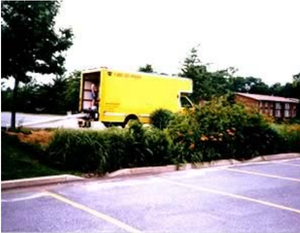
Bioretention areas can be used in parking areas to collect and treat storm water (Source: University of Maryland, 2000)
