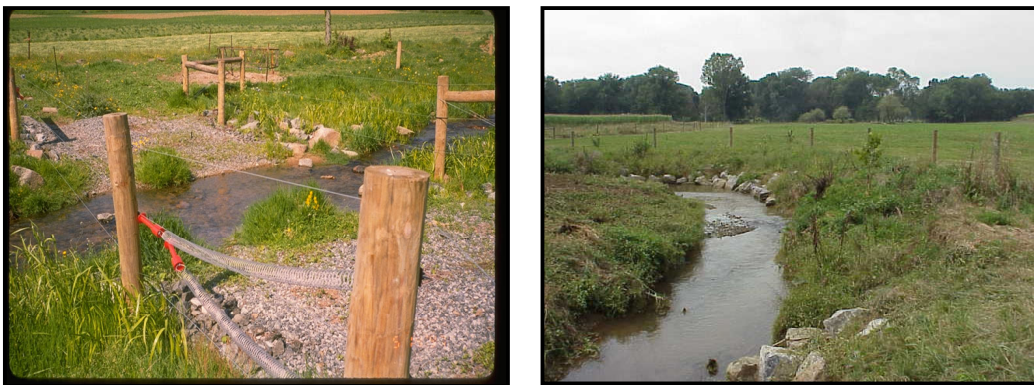
Figure 1.4.6-8 Farmers Installing Cattle Crossings (left) and Streambank Fencing with Riparian Buffers (right) to Limit the Impacts of Livestock on Streambanks and Filter Runoff from Pastures in Berks County.
