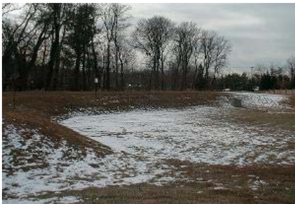
A dry extended detention pond is designed to temporarily detain runoff during storm events
