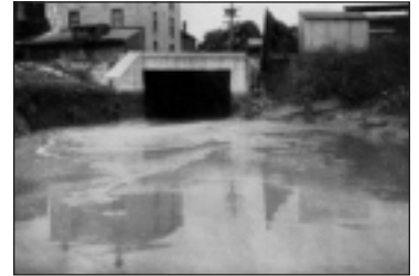
Frankford Creed Wakeling Street Sewer 1914.
