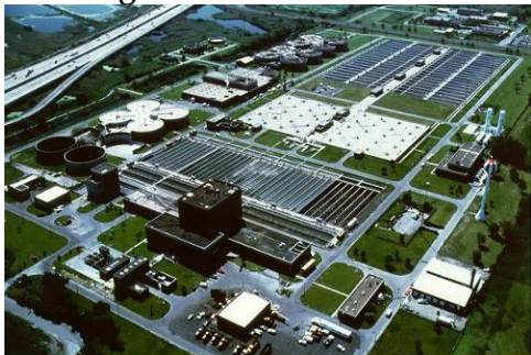
Figure 4-27 Municipal Wastewater Treatment Plant
