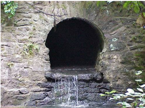
Figure 4-25 Stormwater Outfall
