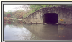
#7 C17 522 MG/yr. Cobbs Creek Beaumont Street and Cobbs Creek 12' x 11.5' outfall
