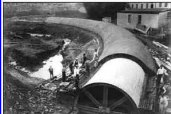
The encapsulation of Mills Creek in 1883. Research credit Adam Levine.
