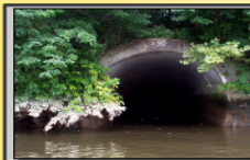
#2 S50 1552 MG/yr. Schuylkill River 43rd Street east of Woodland Avenue Mill Creek 20' x 20' outfall
