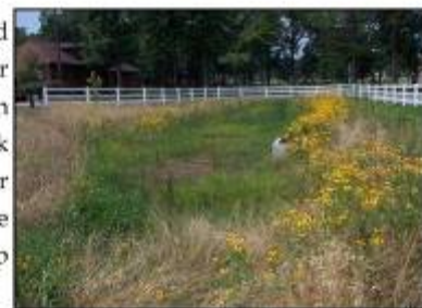
Naturalized stormwater detention basin at Black Rock in Upper Providence Township
