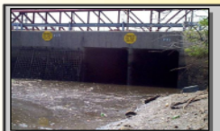
#5 F21 805 MG/yr. Frankford Creek Walking Street northwest of Creek Basin Twin outfall 10.5' x 9.5'
