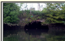
#10 D45 307 MG/yr. Delaware River Laurel Street and Delaware Avenue 14.5' x 10' outfall
