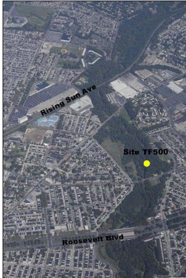
Figure 6-8 Oblique Aerial Photograph of site TF500 and Vicinity
