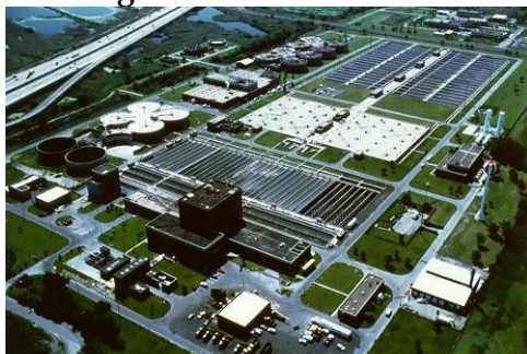
Figure 4.18 Municipal Wastewater Treatment Plant
