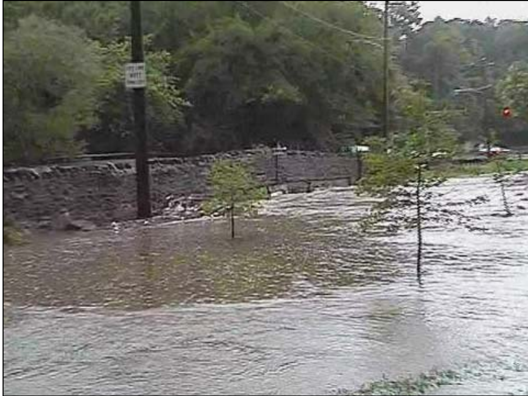
Figure 4.44 Adams Avenue during August 1, 2004 Storm
