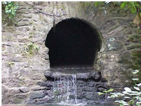
**Figure 4-23 Stormwater Outfall**
