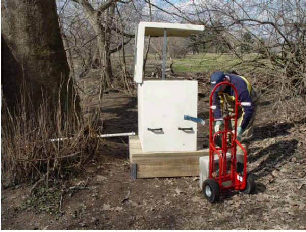
Figure J-11 Automated Water Sampler Installation
