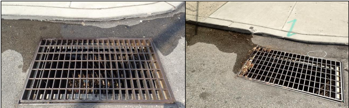
Figure 3-29: Inlet Modification, Before (left) and After (right)
