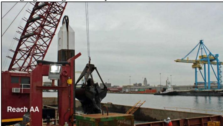
Figure 4.1 Dredging of the Federal Navigation Channel Adjacent to Camden, New Jersey (USACE)
