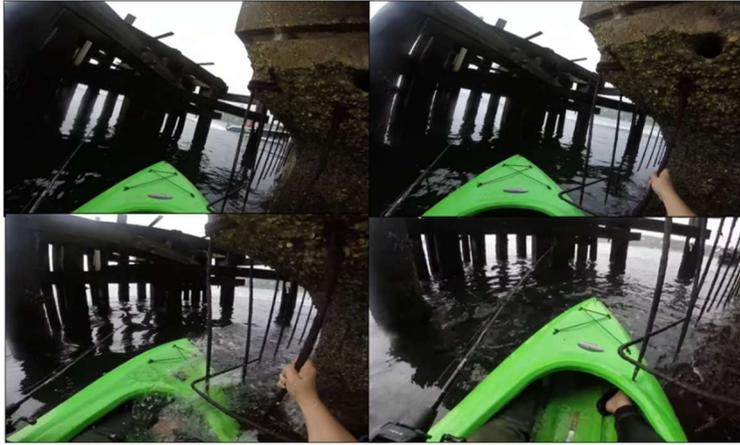
**Figure 6.5 Kayak Pierced by Exposed Rebar from Bridge (Youtube, That Fishing Guy)**
