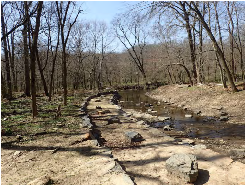
Photograph 2: Boulder terraces following construction at Paul's Run, Philadelphia, PA. Source: PWD.
