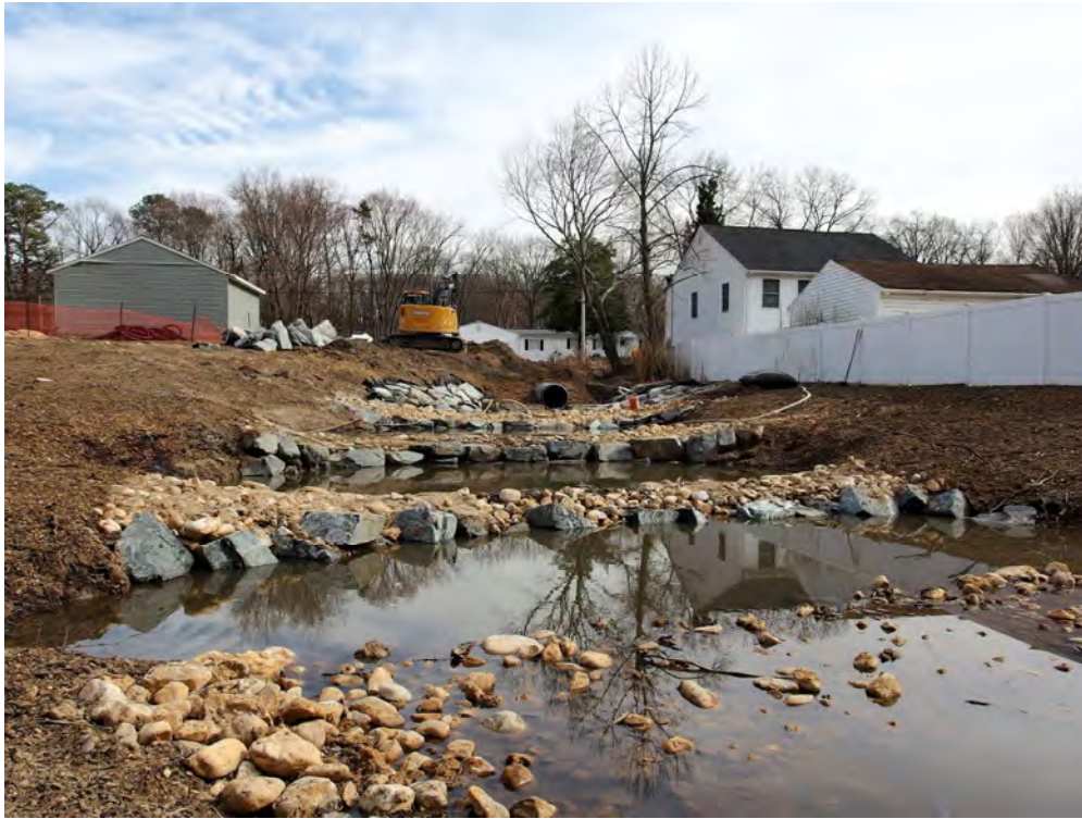
Photograph 1: Regenerative step pool storm conveyance during construction. Source: JMT.
