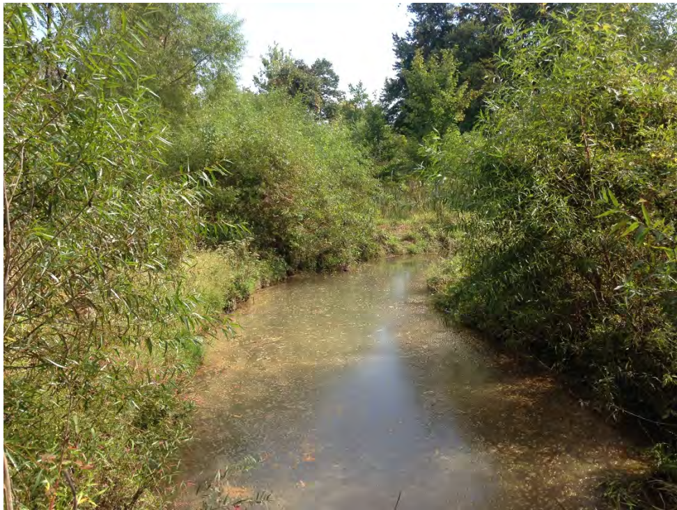
Photograph 2: Pole plantings following construction at Kitten Branch, Anne Arundel County, MD. Source: JMT.
