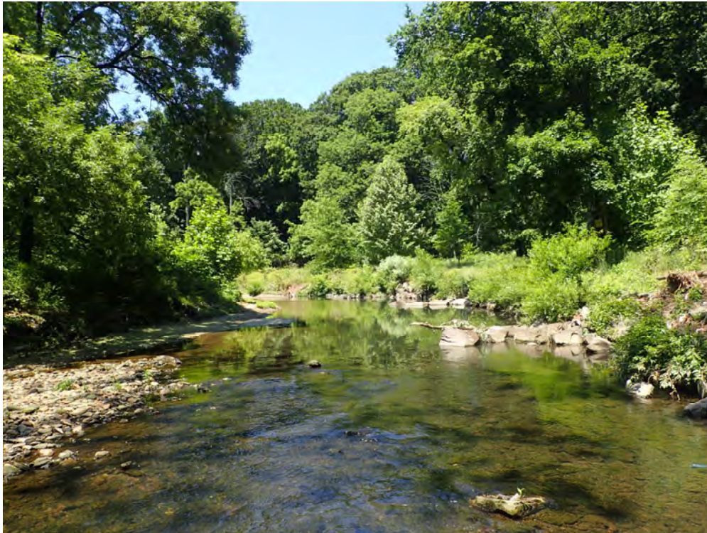
Photograph 2: Bendway weir following construction at Whitaker Avenue, Philadelphia, PA. Source: PWD.
