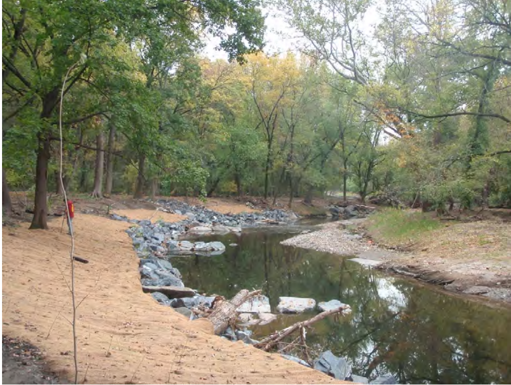
Photograph 1: Bendway weir during construction at Whitaker Avenue, Philadelphia, PA. Source: PWD.
