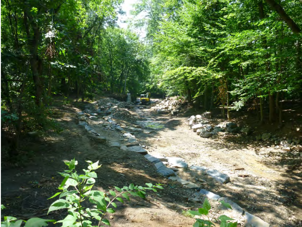
Photograph 1: Boulder terraces during construction at Paul's Run, Philadelphia, PA. Source: PWD.
