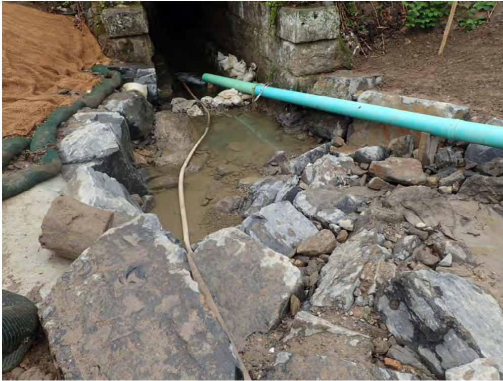
Photograph 1: Boulder cascade during construction at Cresheim Creek, Philadelphia, PA. Source: PWD.
