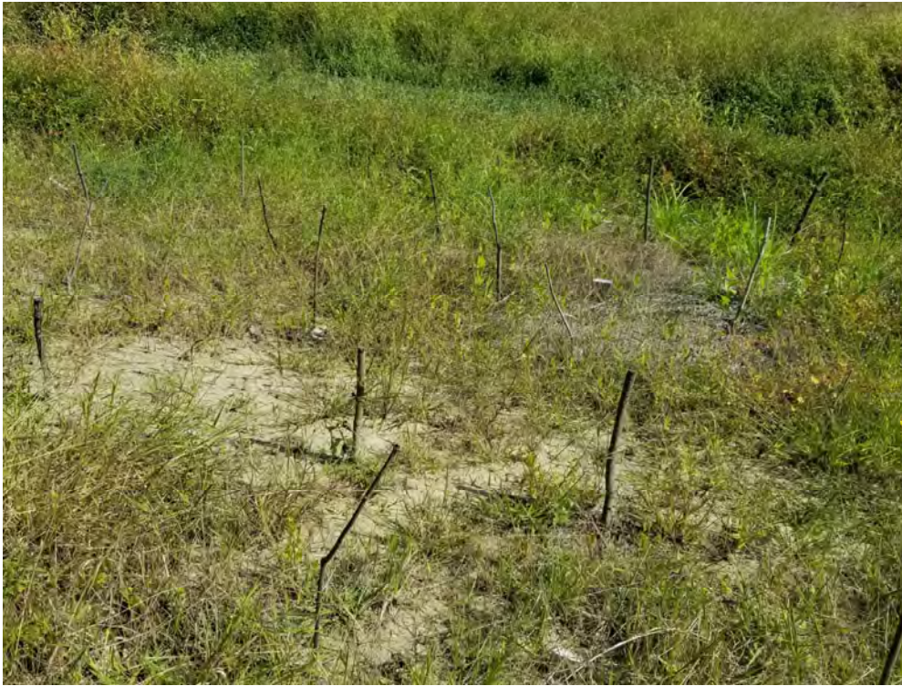
Photograph 1: Live stake plantings during construction. Source: JMT.
