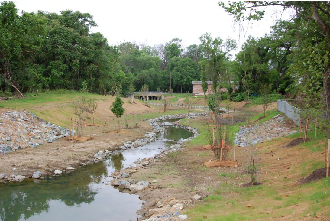
Photograph 2: Riprap revetment following construction at Nash Run, Washington, DC. Source: JMT.
