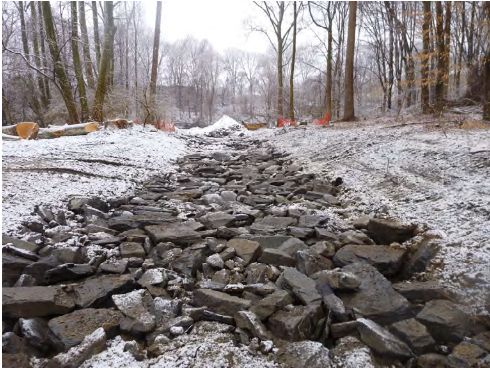
Photograph 1: Engineered riffle during construction at West Branch Indian Creek, Philadelphia, PA.
