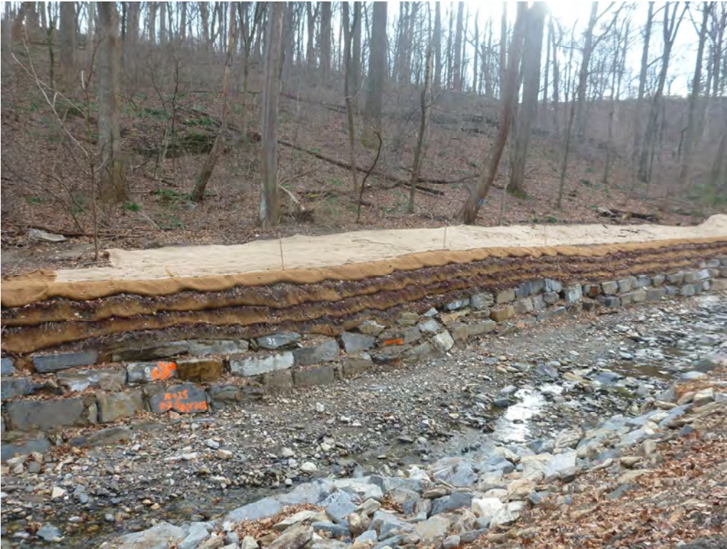
Photograph 1: Soil lifts during construction at Gorgas Run, Philadelphia, PA. Source: PWD.
