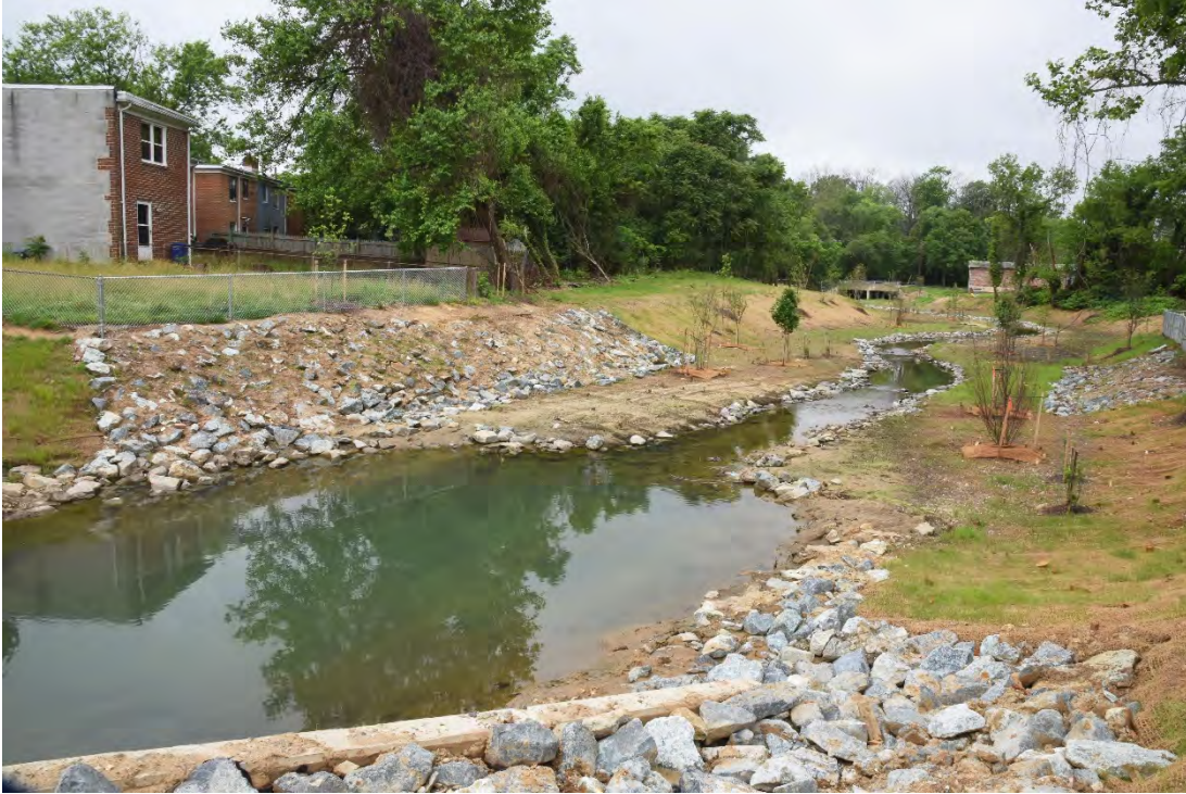
Photograph 1: Riprap revetment following construction at Nash Run, Washington, DC. Source: JMT.
