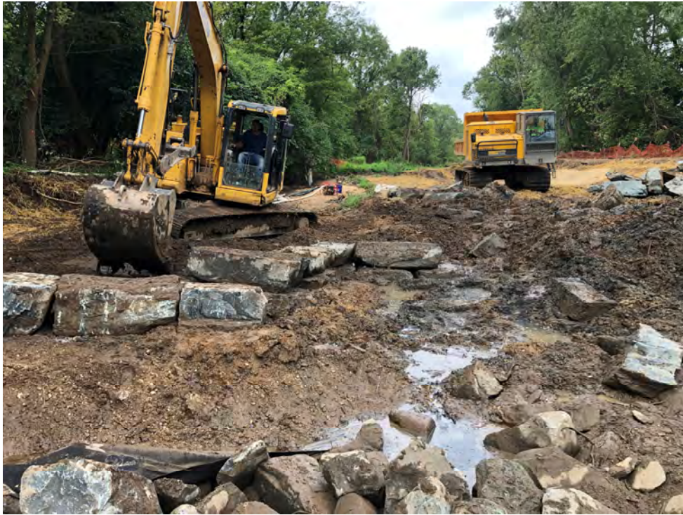
Photograph 1: Offset cross rock vane during construction at UNT to Patapsco River, Baltimore County, MD. Source: JMT.
