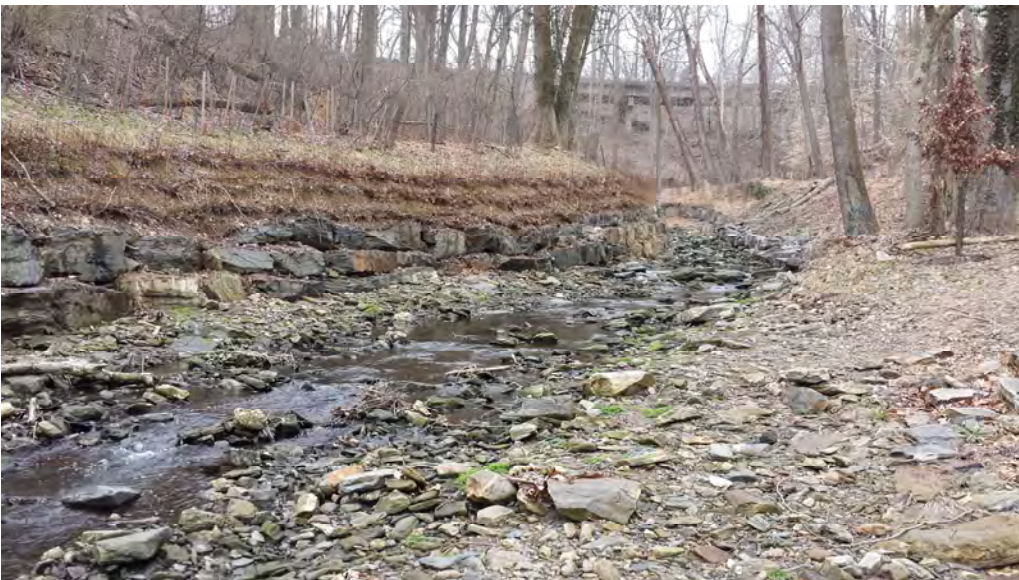
Photograph 2: Soil lifts following construction at Gorgas Run, Philadelphia, PA. Source: PWD.
