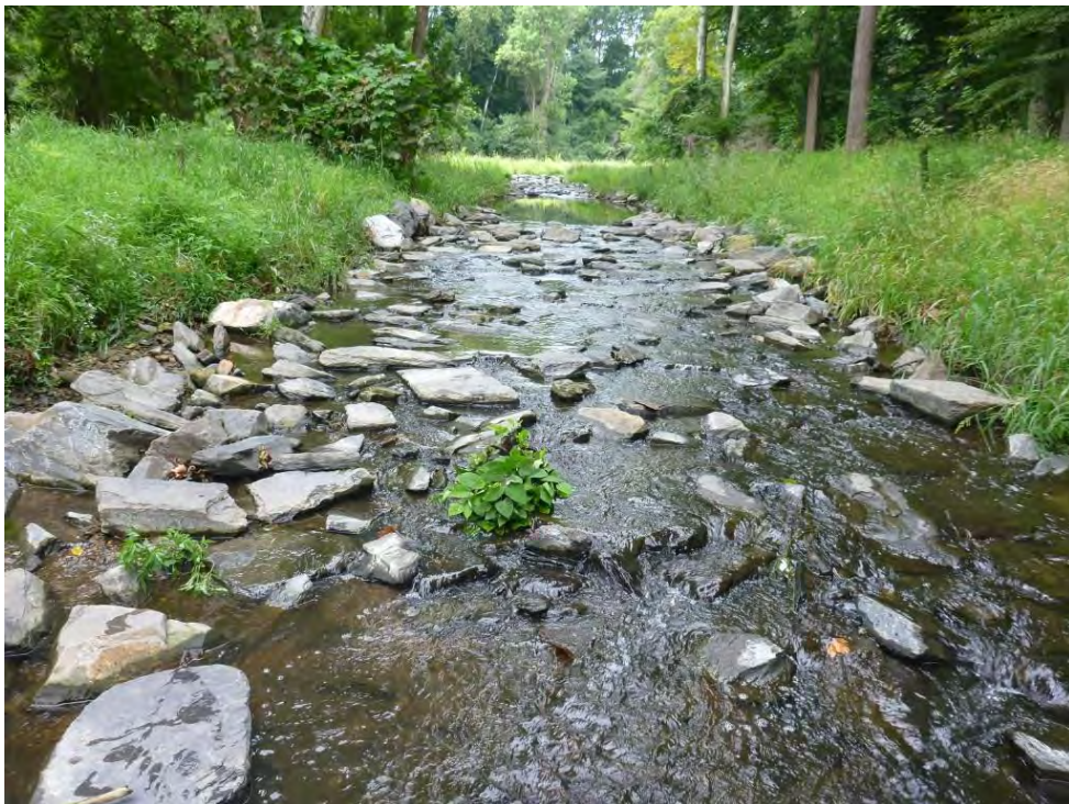
Photograph 2: Engineered riffle following construction at West Branch Indian Creek, Philadelphia, PA.
