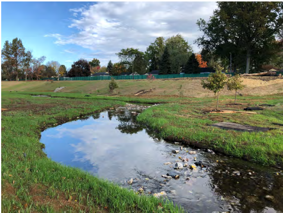
Photograph 2: Typical pool cross section following construction at Stickney Creek, Cuyahoga County, OH. Source: JMT.
