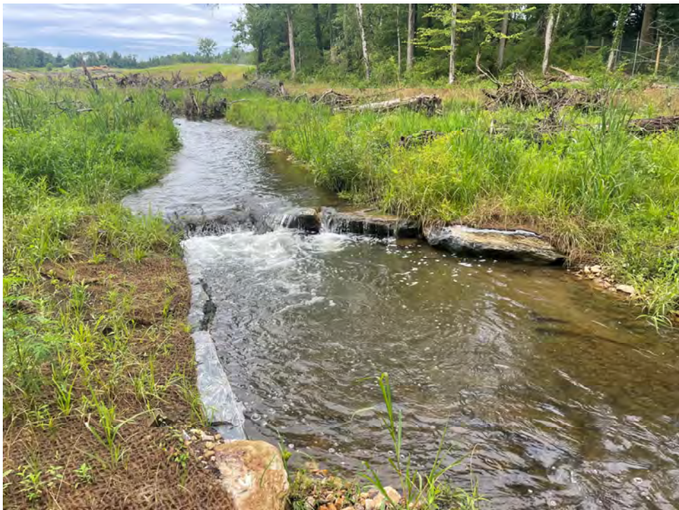
Photograph 2: Offset cross rock vane following construction at Jones Falls, Baltimore County, MD. Source: JMT.
