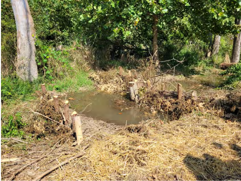
Photograph 1: Beaver dam analogs during construction at Beaver Creek, Washington County, MD. Source: JMT.
