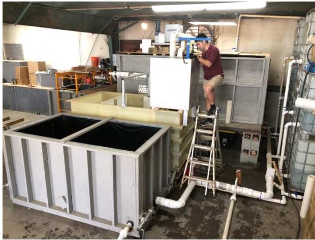
Inlet Basin Resting on Weir Box
