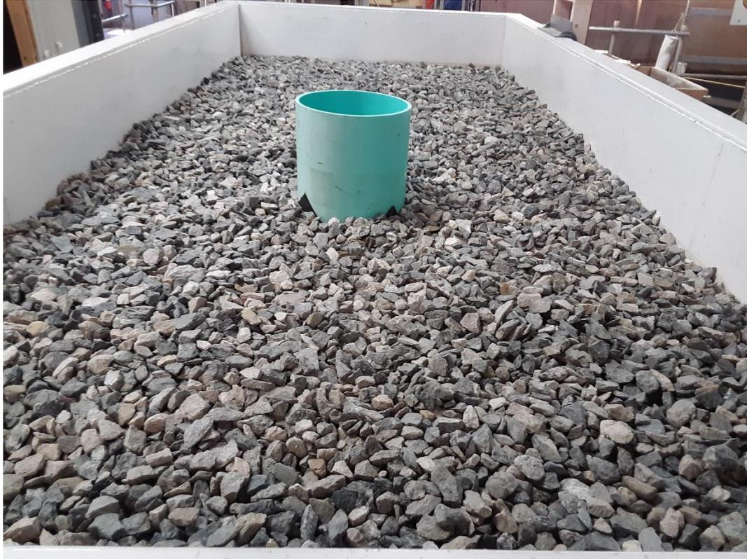
**Figure 6 Installed R-Tank Treatment Row System**
